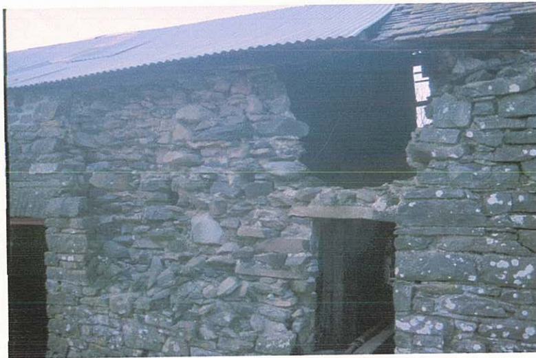
Plate 5: Detail of Farm Building Showing Collapsed Masonry.
