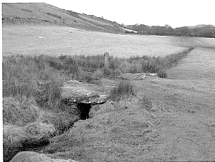
Prn 45798 – the culvert and leat exiting the mine processing complex
