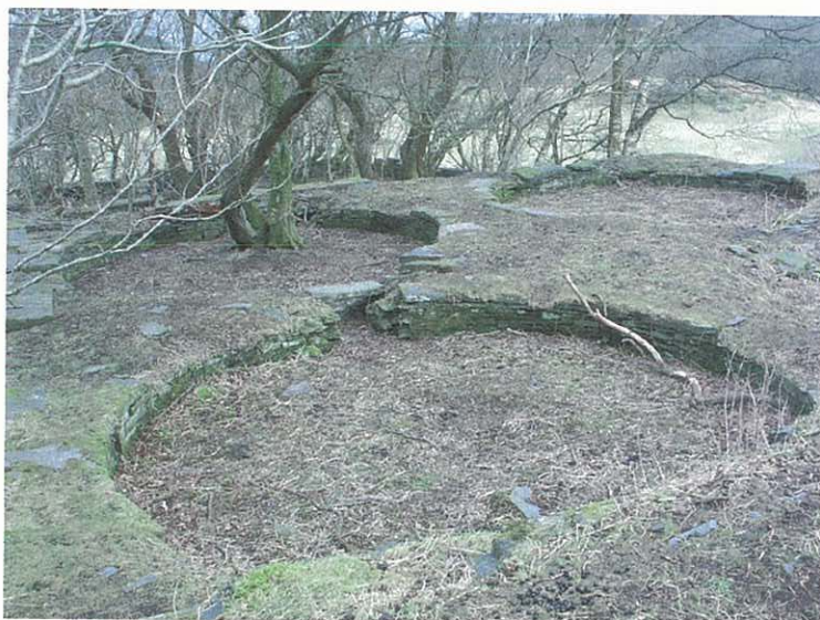
Prn 45792 – a system of four buddles, with interconnecting sluices
