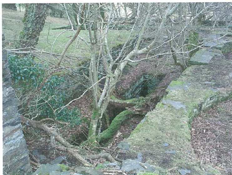
Prn 45793 – the wheel pit which provided power for the buddles
