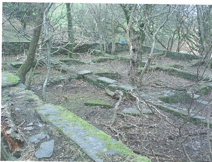
Prn 45794 – a series of 18 settling tanks, rather overgrown with trees.
