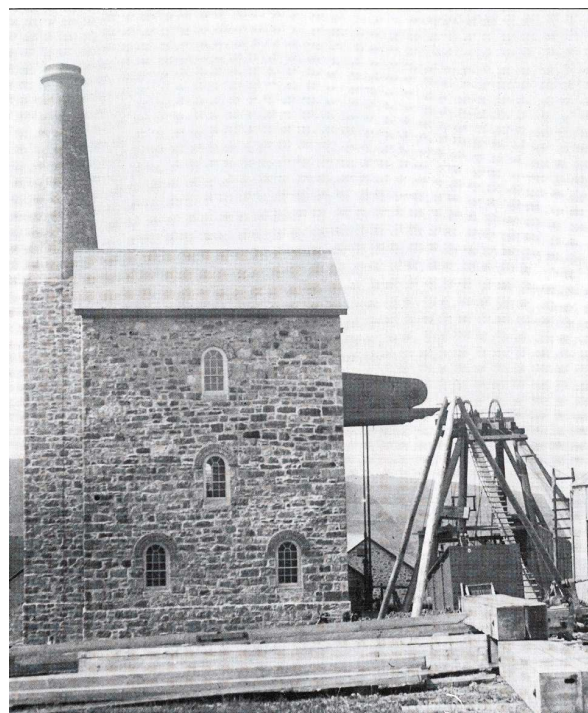
Plate 3- a complete Cornish engine house- newly erected at Phoenix Mine in 1907 with shaft timbering in foreground ready to be fitted (Stanier 1988: 19).
