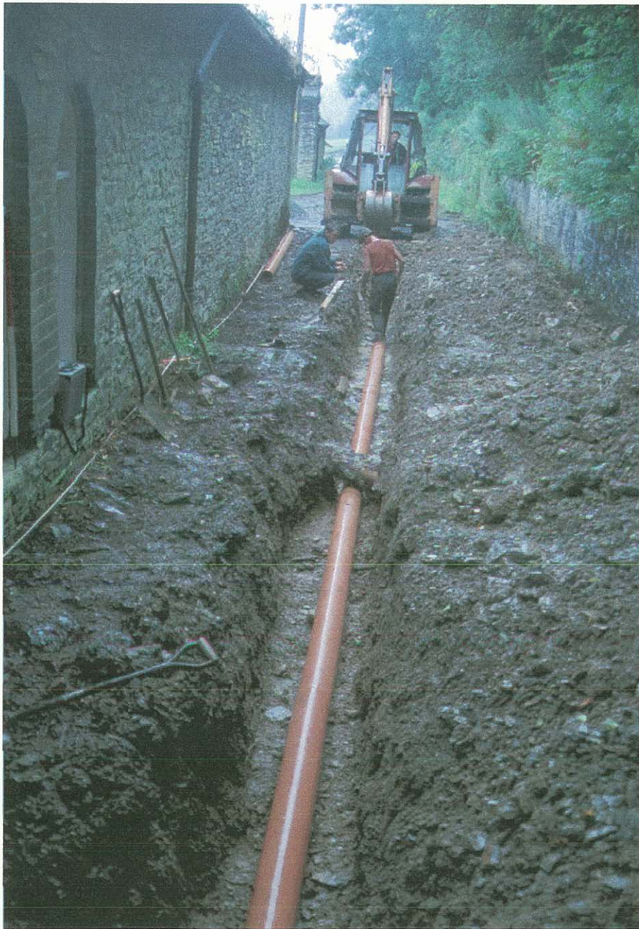
Photograph 2. Working shot during excavation of sewerage pipe trench on north-west side of stable block.
