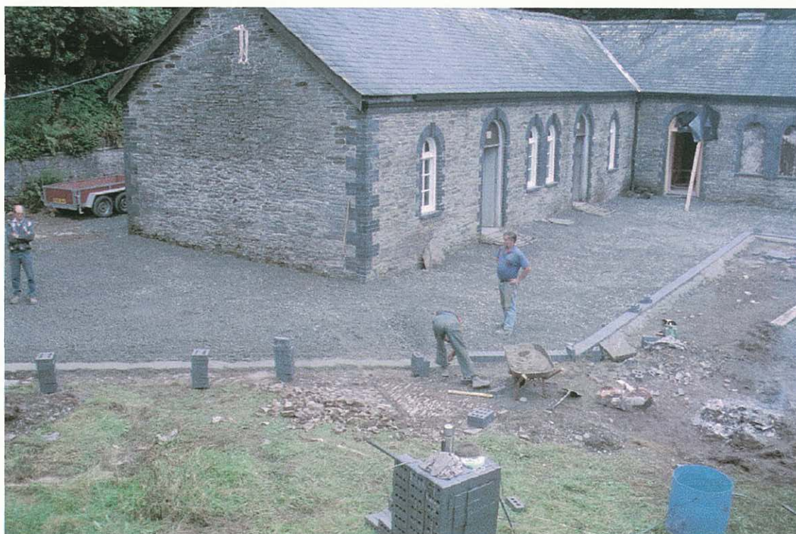
Photograph 6. View of stable courtyard looking north during laying of stone apron. Pitched cobbling (O) in foreground.
