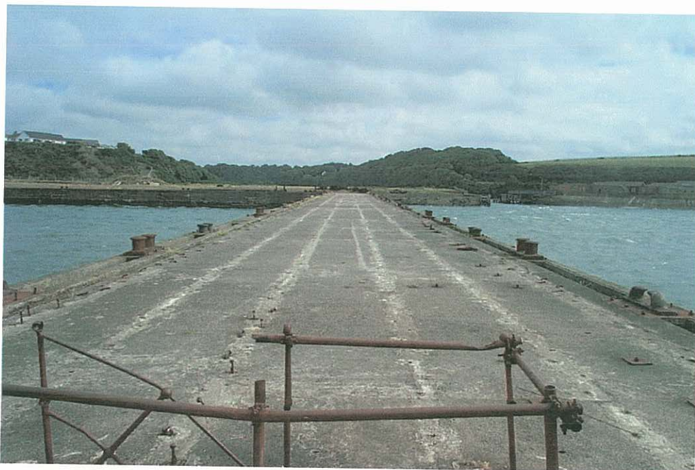
Plate 4: Ward's Yard Pier (PRN 34962). A view north along the pier, constructed during the 1930s, showing the ghosts of the railway lines that once took the scrap metal away from the ships being dismantled along either side of the pier. Several photographs held in the Milford Haven Museum show the pier under construction.
