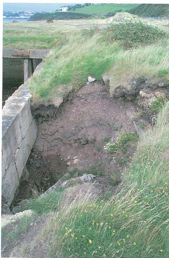
Plate 2: eroded section behind sea wall showing the dumps of material for the made ground on the west bank of the pill. The photograph shows the landward end of the pier (PRN 34962) and is looking west across the site of the former RNAS airship station (PRN 28667).
