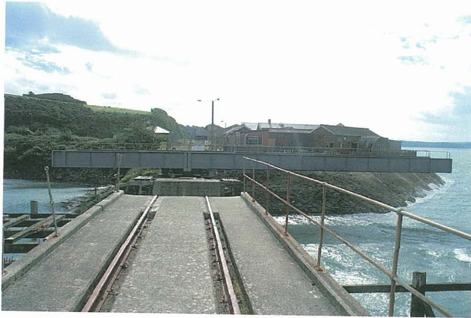
Plate 3: Swing bridge PRN 8787. The bridge is likely to be renovated during the proposed development. The current bridge, probably built in 1939, replaced the original 19 th century swing bridge.
