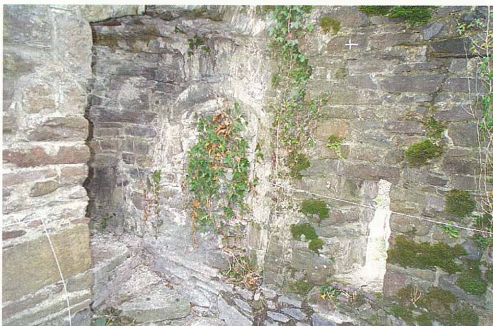
Photo 24 – The blocked entry into the former turret from the south side of the gatehouse first floor, facing southeast. The area to the left has been damaged and altered (see Fig. 24b)
