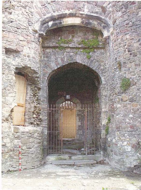
Photo 17 – The gate-passage entry from the outside, facing east, before excavation. The early 15 th century dressings can be seen. The flanking opening in the north tower has been unblocked (see Fig. 15)
