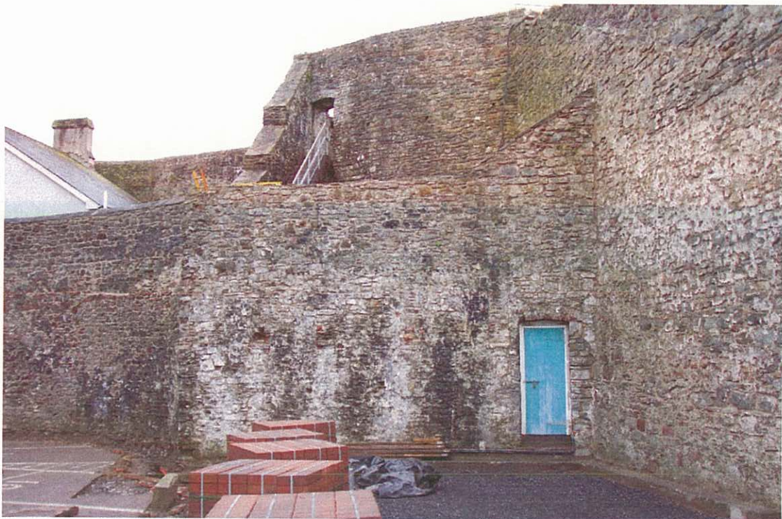
Photo 4 – The exterior of the forebuilding east wall, showing chases for the gaol-phase passage arches. The shell-keep, and its entry, can be seen beyond (see Fig. 4)
