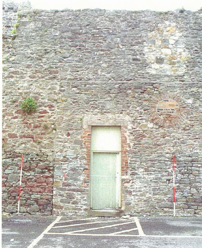
Photo 34 – The west face of the infirmary east wall, showing the medallion and the infill of the ?first floor chase (see Fig. 34)
