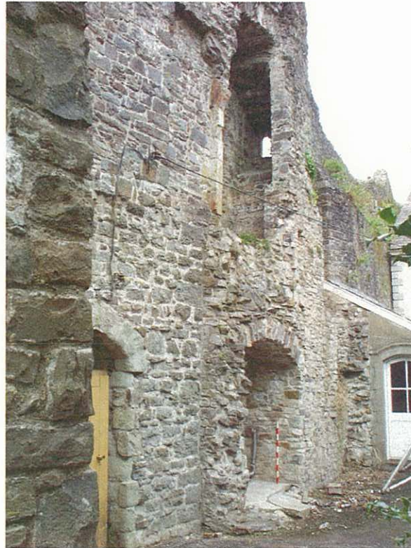
Photo 15 – The gatehouse east face, facing northwest. The gaol-phase infill and entry are to the left, and to the right are the scar of the rear section north wall and the doorway to the west curtain wall-walk (see Fig. 17)
