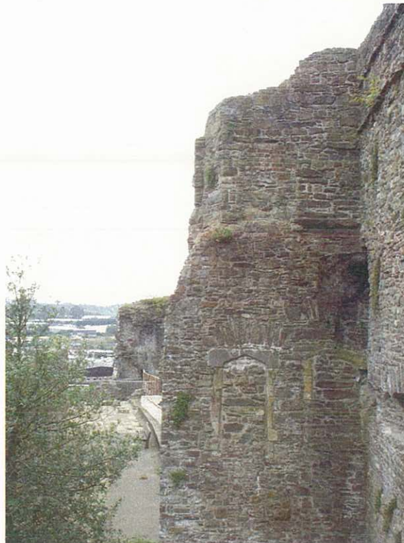
Photo 16 – The remains of the gatehouse rear section south wall, facing south, showing the blocked first floor entries, and secondary entry (see Fig. 18)
