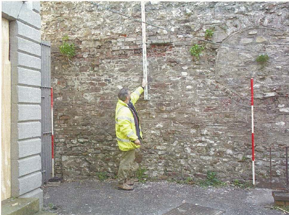
Photo 34 – The west face of the infirmary east wall, showing the medallion and the infill of the ?first floor chase (see Fig. 34)
