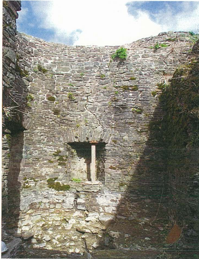
Photo 25 – The gatehouse first floor facing north, showing the blocked north tower window opening, and part-excavated ground floor infill below it (see Fig. 24c)
