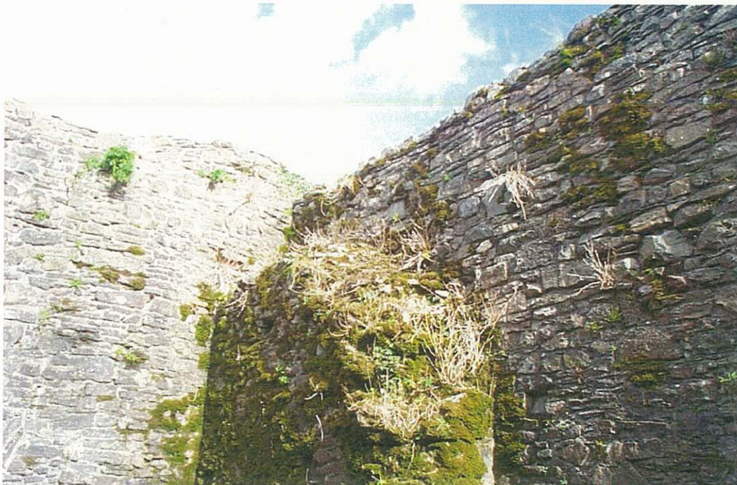
Photo 26 – The northeast corner of the gatehouse first floor, facing northeast, showing the coped vaulting over the mural passage to the west curtain wall-walk (see Fig. 24c and d)
