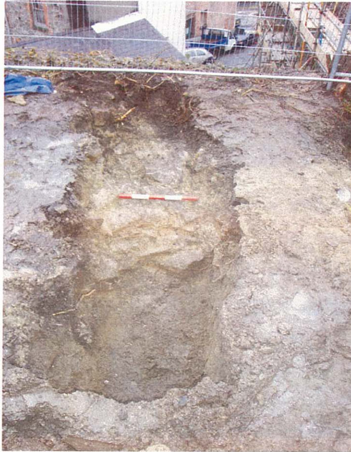
Photo 10 – The ?c.1901 buttresses against the internal face of the northern shell-wall, revealed by construction trenches 27 - 29, facing northeast (see Fig. 8)
