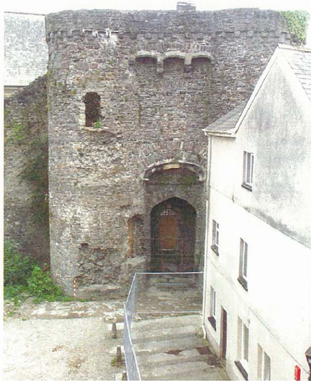
Photo 14 – The gatehouse from the south, after the demolition of the Rugby Club. The truncated west curtain wall, and the remains of the turret in its angle, can be seen, and the large area of robbing and infill in the central lower half (see Fig. 16)
