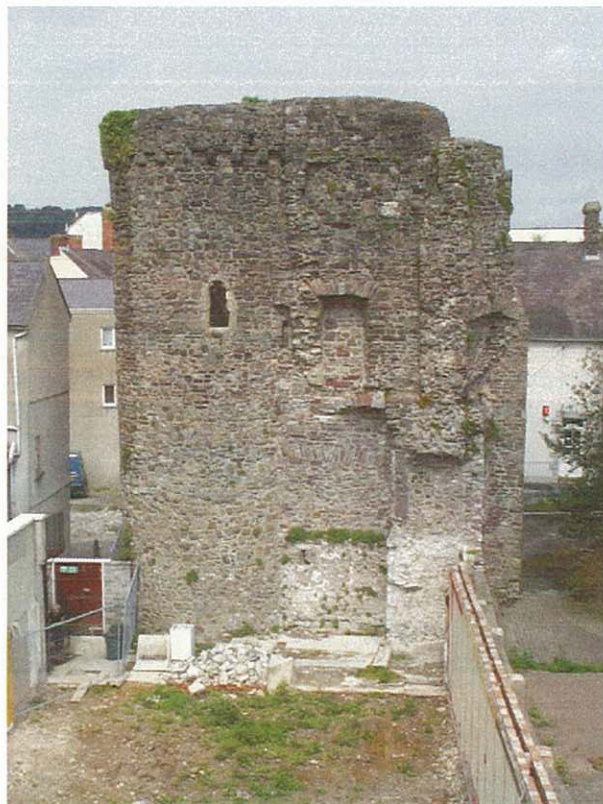
Photo 14 – The gatehouse from the south, after the demolition of the Rugby Club. The truncated west curtain wall, and the remains of the turret in its angle, can be seen, and the large area of robbing and infill in the central lower half (see Fig. 16)
