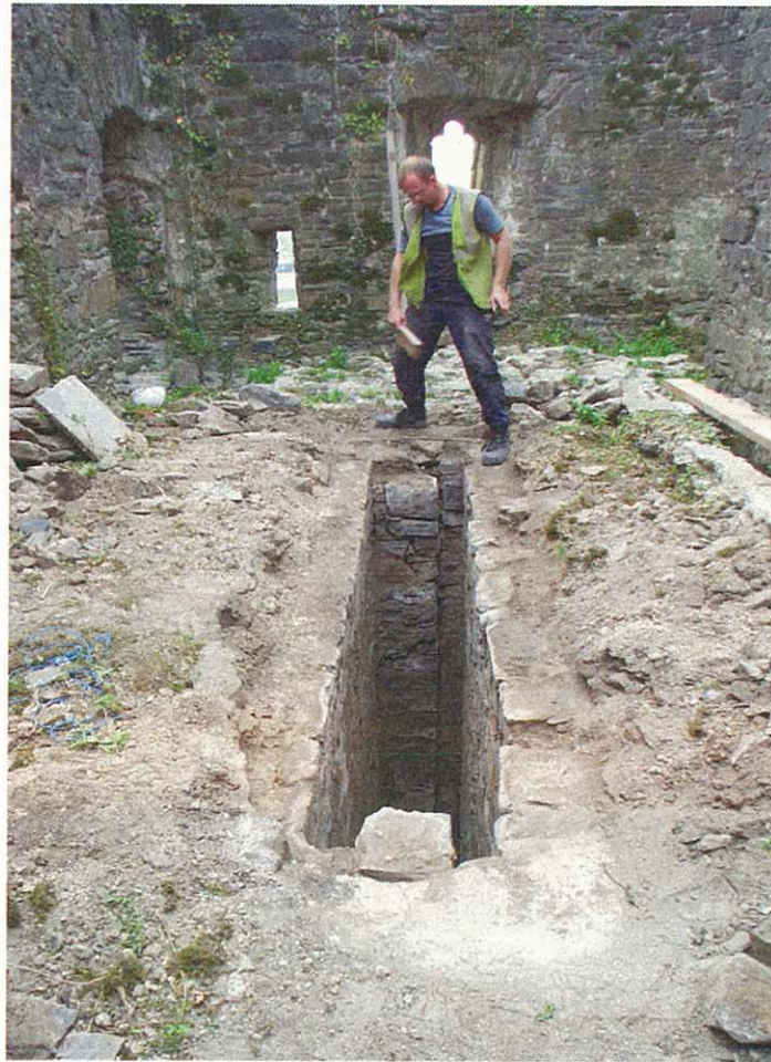
Photo 27 – The gatehouse first floor, facing south, during removal of later slabbing from over the portcullis slot (see Fig. 23)
