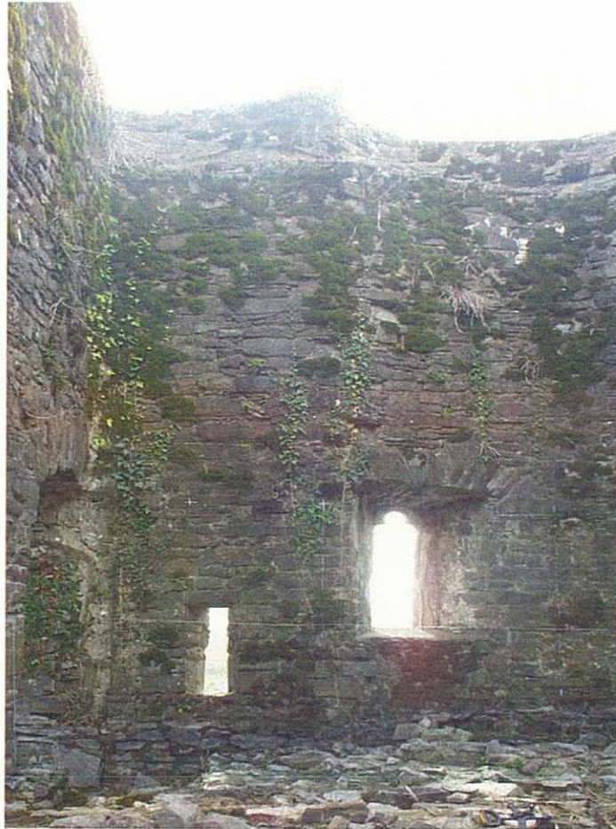
Photo 23 – The gatehouse first floor, facing south, showing the surviving 15 th century surround in the window opening, and the top of the ground floor infill (see Fig. 24b)
