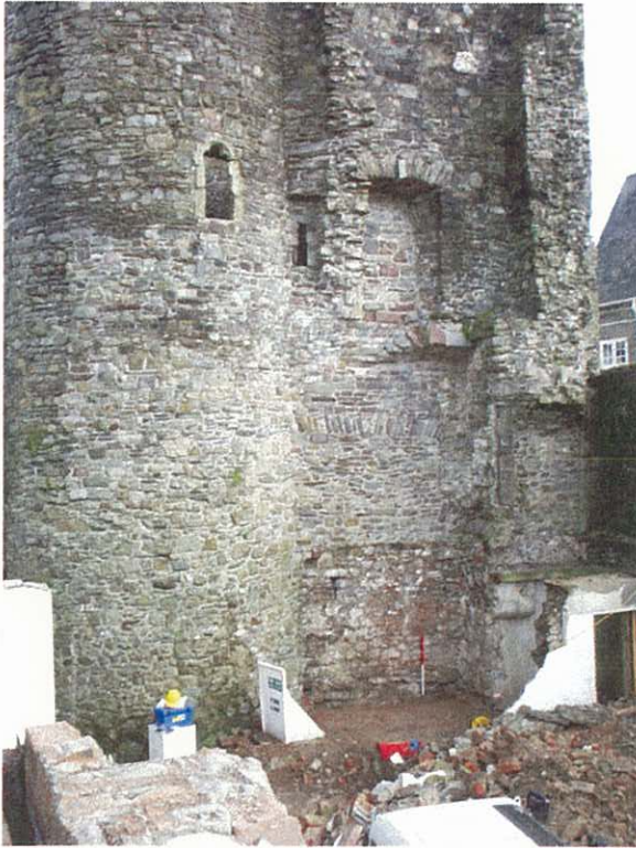
Photo 1: Gatehouse south site with render partly removed, view NNE, scale 1m
