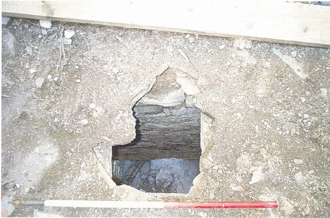
Photo 3: Gatehouse collapse into passageway, view W, scale 1m
