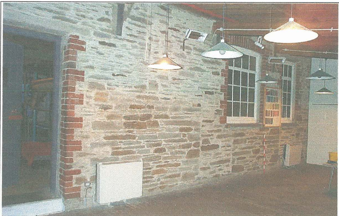
Plate 12: Covered yard, first floor Room N south wall with 1902 doorways blocked/alterd in 1919-20
