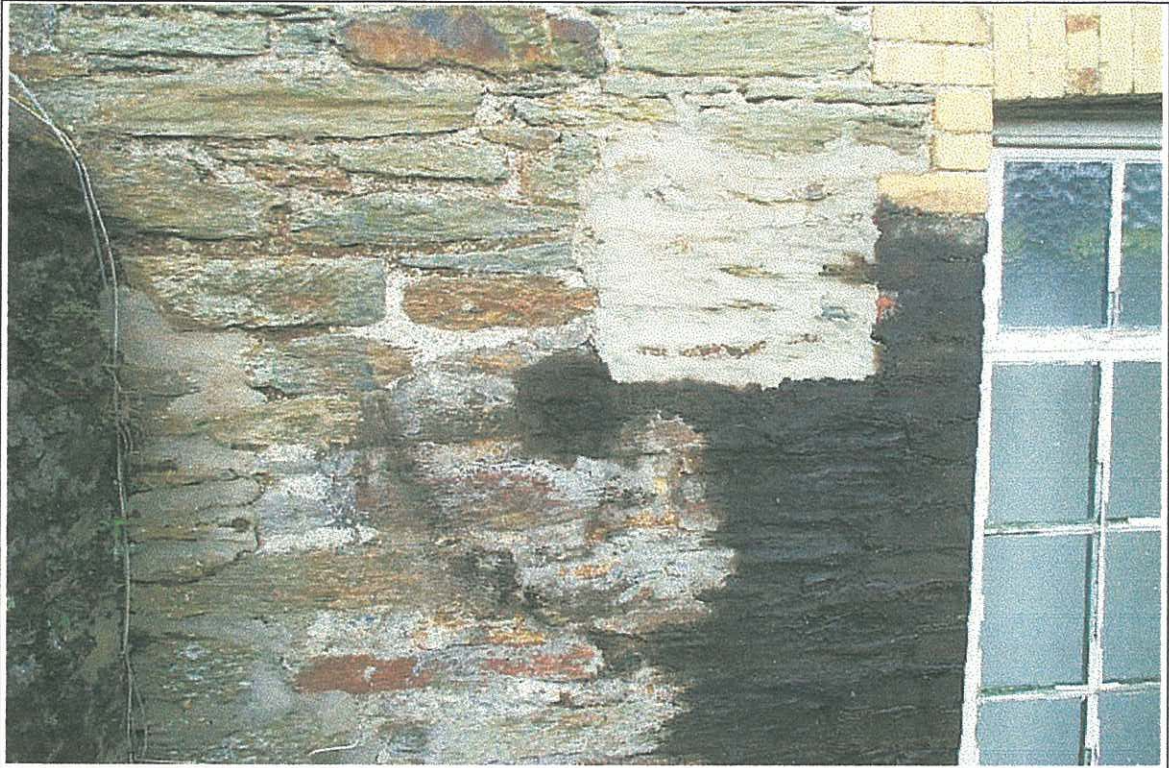
Plate 15: Scar of drive wheel on exterior of southeast elevation
