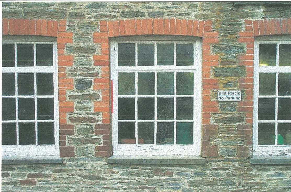
Plate 16: Detail of brick window surround of ground floor southwest wall of Mill 1
