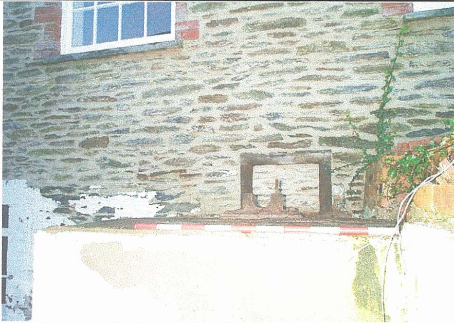
Plate 13: Open yard, looking west at Mill 2, showing external machine bearing
