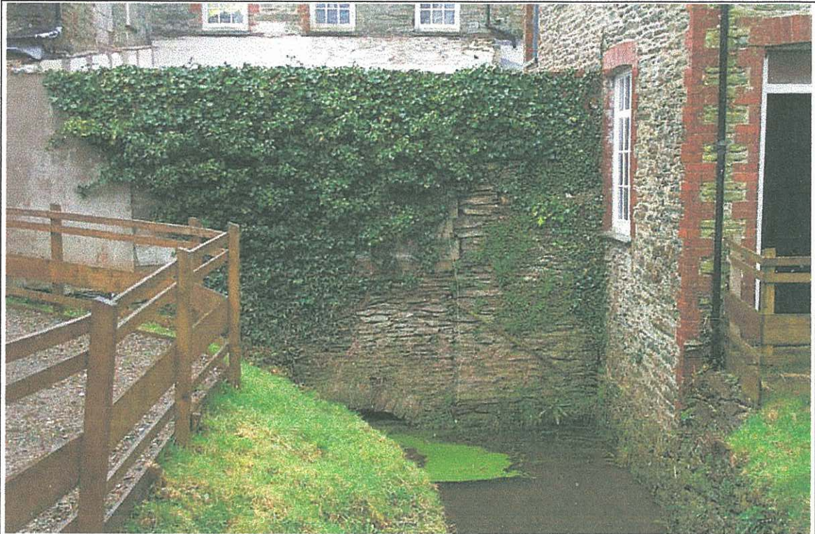
Plate 17: Stonework above tailrace. Possibly from the Phase 1, pre-1888 mill.
