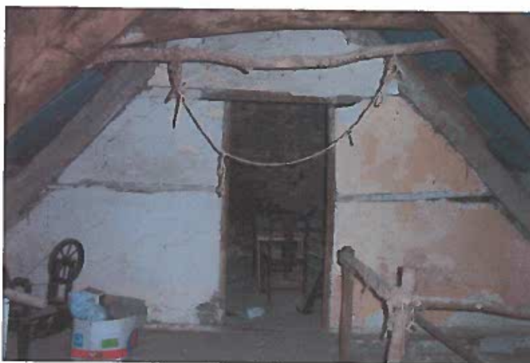
Plate 6. The upper storey of the old farmhouse (PRN 47805). An interior partition wall. The plaster is beginning to fall off at the base of the left door post, revealing the wattle structure of the wall.
