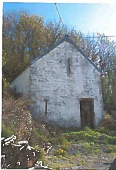
Plate 1. The south elevation of the barn (PRN 47800) showing the narrow ventilation slits which splay to a wider opening on the inside.
