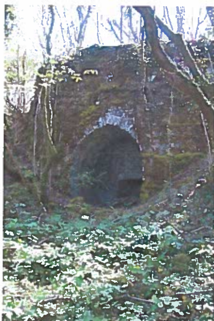
Plate 7. The well preserved drawing arch of a limekiln (PRN 27778) with the kiln eye visible inside.
