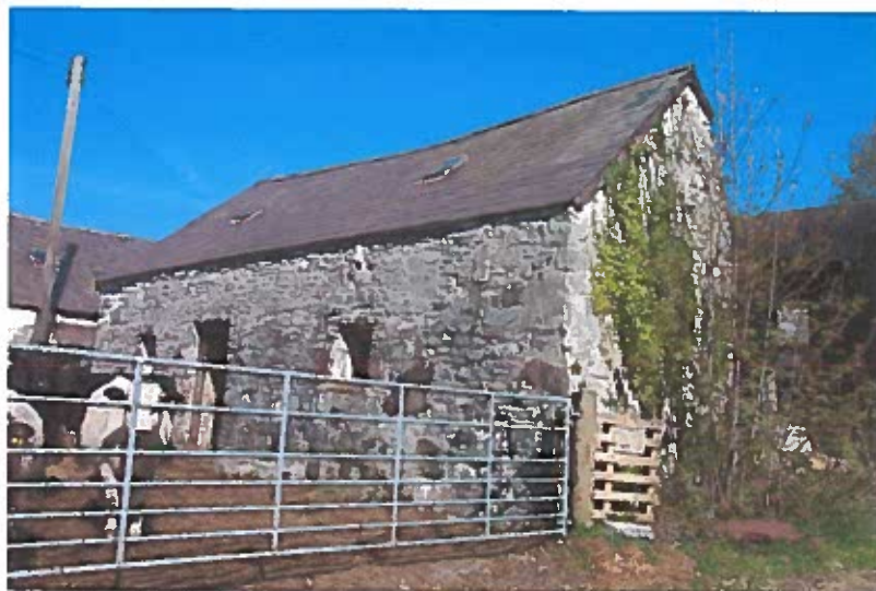
Plate 3. The cowshed (PRN 47802) which was converted from a house or cottage (PRN 47807). The southeast corner (in the foreground) has been modified to incorporate what was previously an external chimney. The south elevation, seen in this picture, gives an impression of what the house may have looked like.
