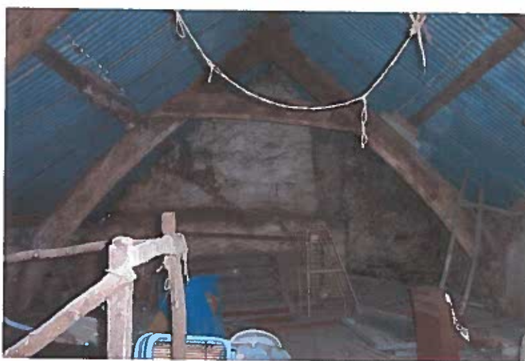
Plate 5. The upper storey of the old farmhouse (PRN 47805.) One of the upper cruck trusses which supported the roof.
