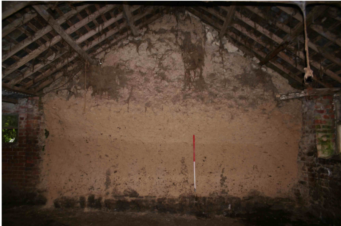
The clom walling demonstrates the constructional sequence, with horizontal building 'lifts' clearly visible
