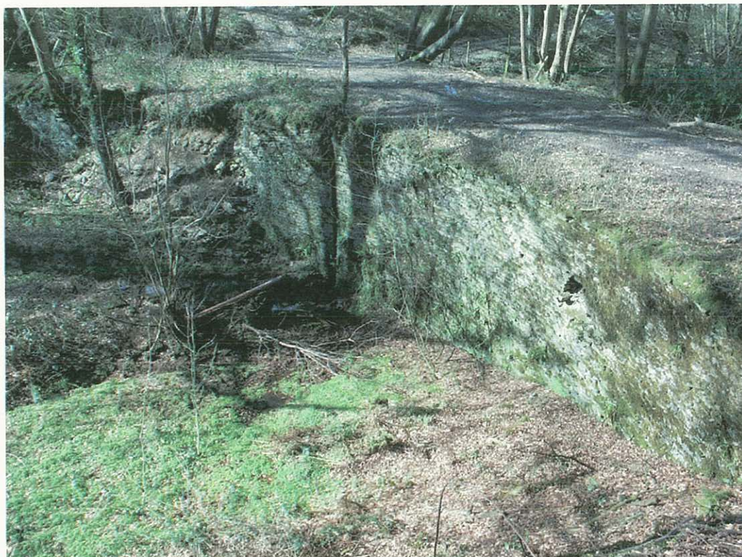
Plate 5 – the south east face of the dam (PRN 44583), showing collapse at the west side.
