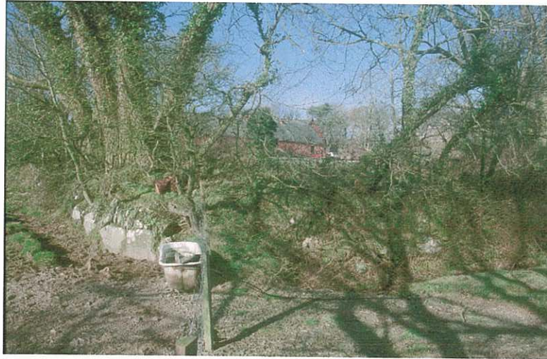
Plate 5: If the long term future of this feature is to be secured, it will be necessary to cut down the trees growing on the retaining bank to prevent further damage to the structure. Depending on the extent to which the bank has been weakened by this tree growth, it may be necessary to remove the stumps and roots and reconstruct the stonework.
