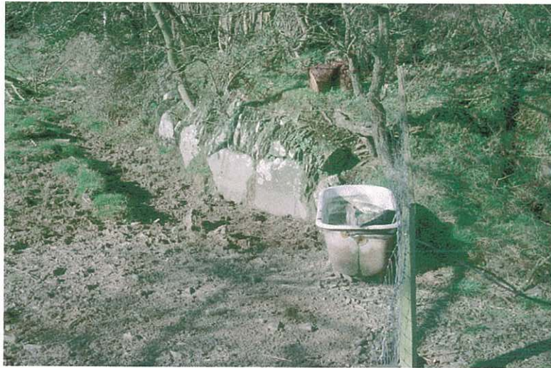
Plate 1: The base of the retaining bank is constructed from impressive stonework, suggesting that this aspect of the feature was intended to be visible. Material that has fallen from the bank could be removed to expose more stonework and to supply stones for making repairs to the structure.
