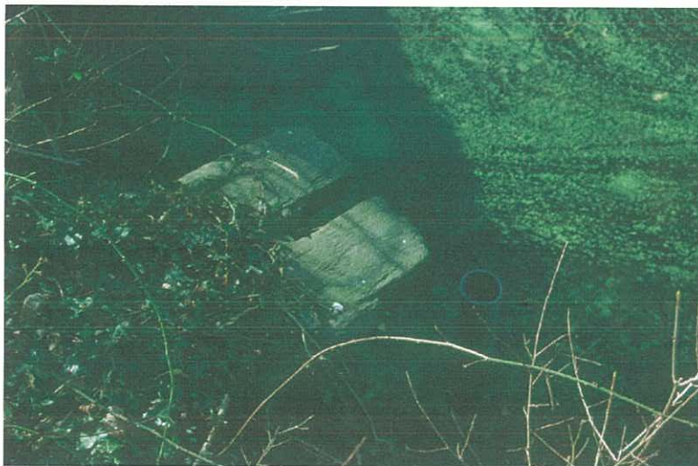
Plate 1: The base of the retaining bank is constructed from impressive stonework, suggesting that this aspect of the feature was intended to be visible. Material that has fallen from the bank could be removed to expose more stonework and to supply stones for making repairs to the structure.
