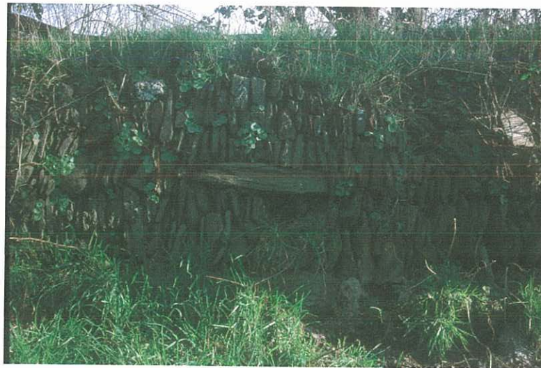
Plate 4: The overflow pipe for the pond, indicating the level to which the water could rise. Larger vegetation that is causing the stonework to loosen should be removed to prevent further weakening of the retaining bank. Stonework should be repaired with the same materials, techniques and pattern as was used in the original construction.
