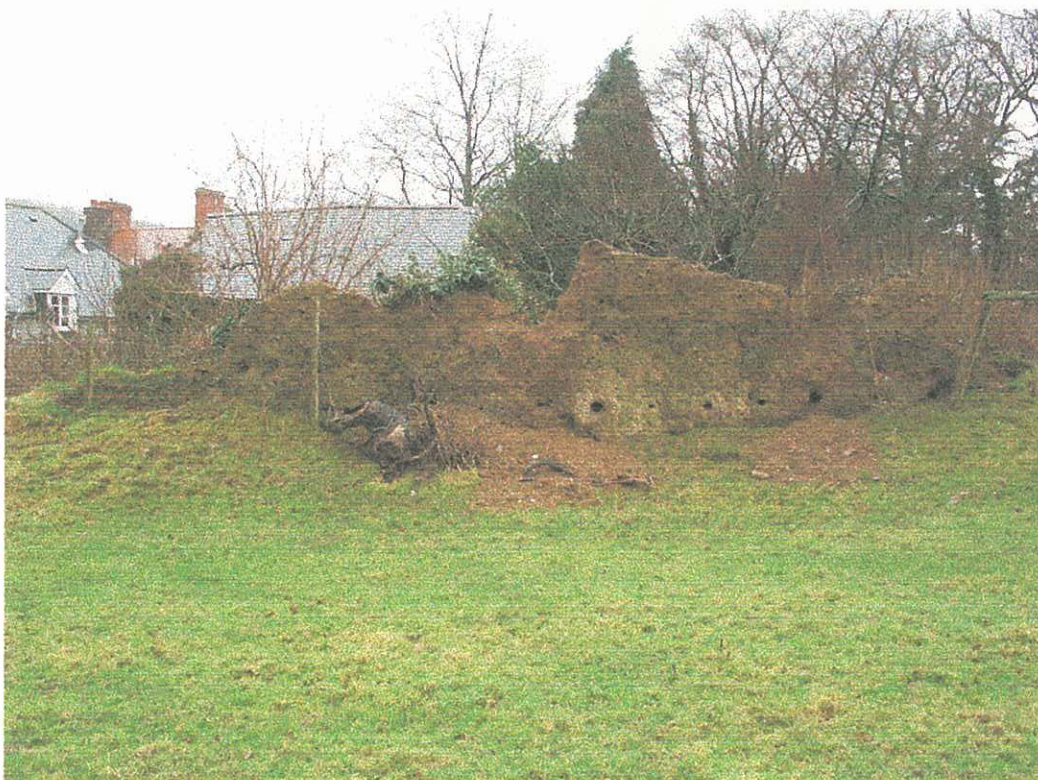
Plate 5 – the remains of a clom or mud wall (PRN 43961)
