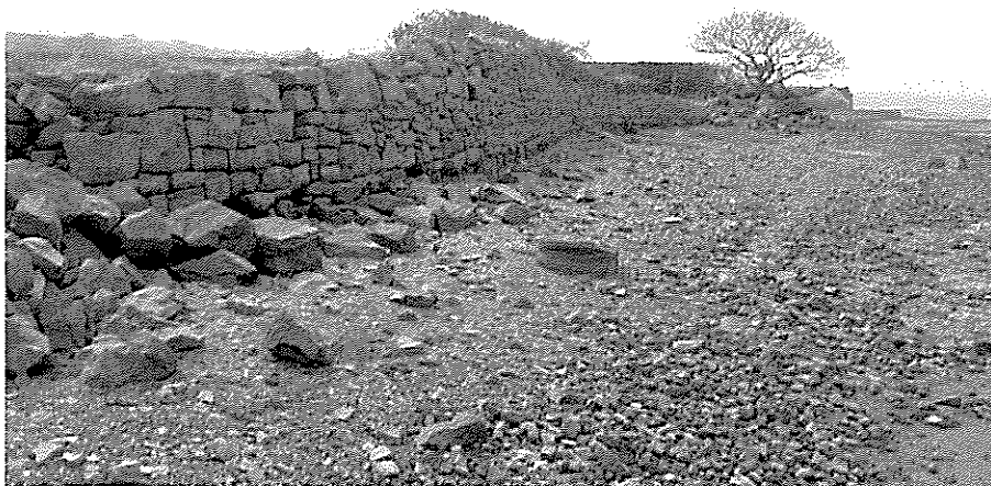
Plate 5 – the partly collapsed sea wall (PRN 35060) looking west.
