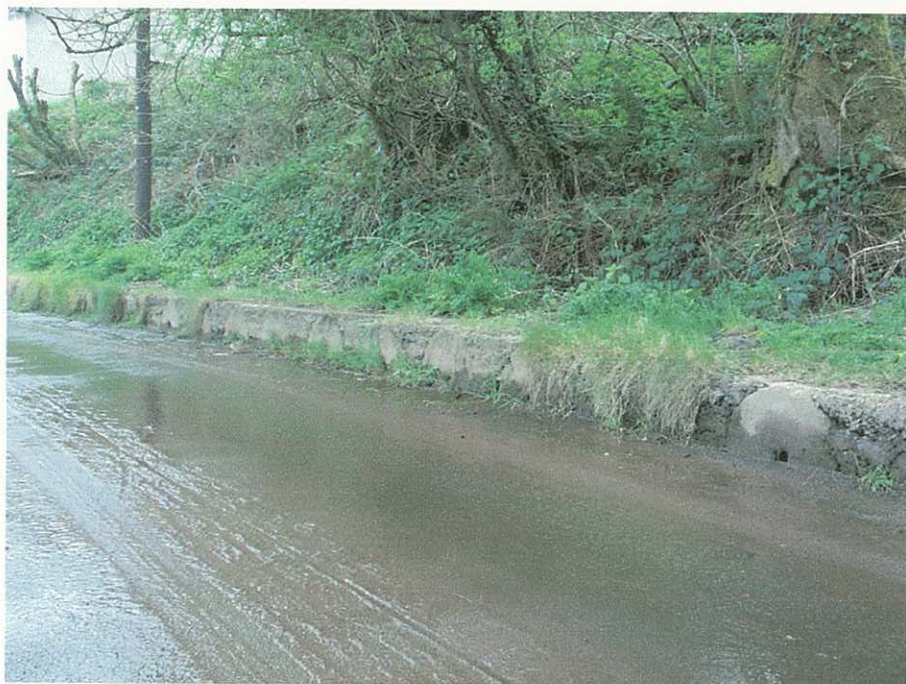
Plate 4 – concrete barbed wire entanglement blocks have been reused to provide a raised walkway
