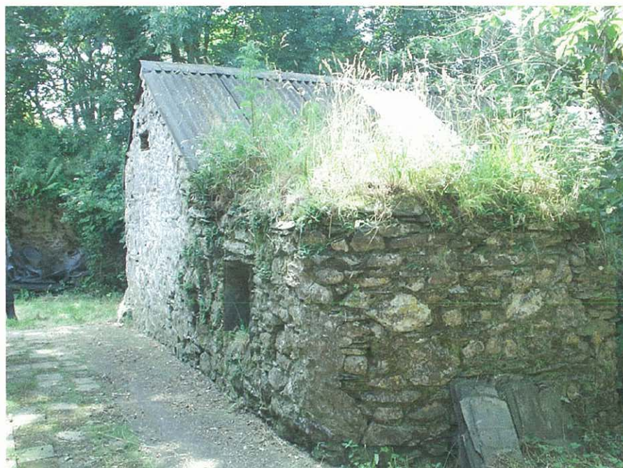
Prn 47749 – the pigsty, with a slate lined feed chute in the yard wall.
