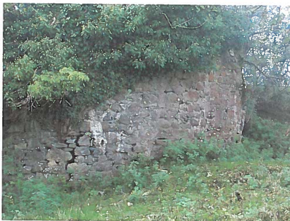
Plate 4: PRN 15967 – Cracking and movement in the north wall of the limekiln. The kiln is a Listed Building Grade II, so Listed Building Consent would be required for any remedial works.
