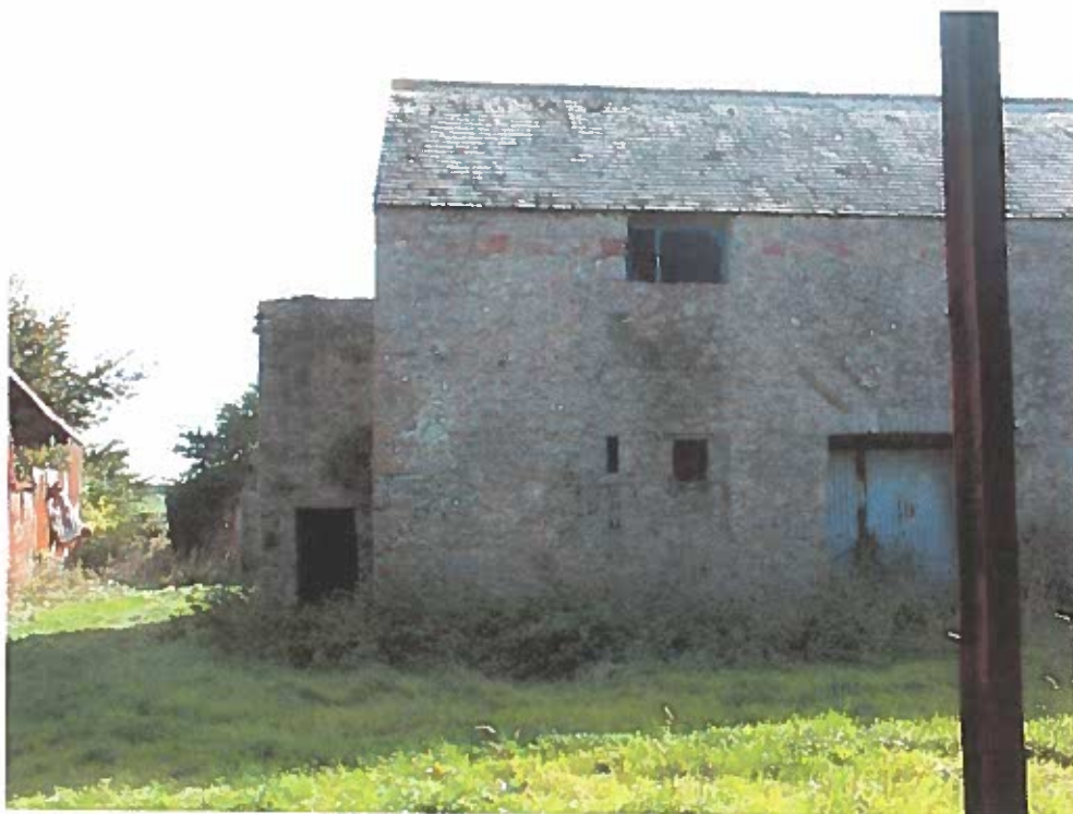
Plate 3: PRN 43614 – 18 th century threshing barn, showing roof scars and rectangular hole for gear from a former horse engine.
