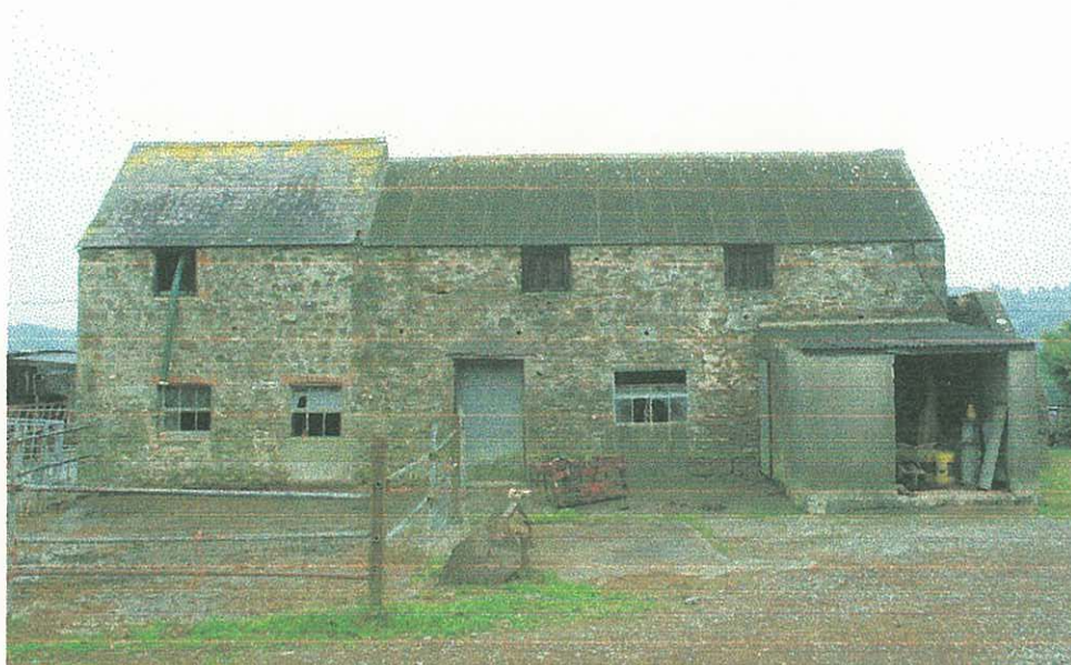
Plate 2 – the cow house (42902) to the south of the farmyard showing its two phases of construction and modernised openings.
