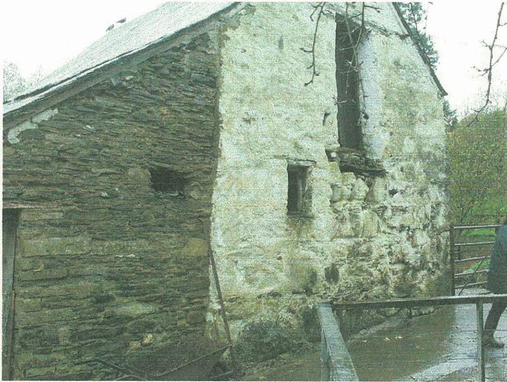
Plate 1: PRN 43769 – stable showing the differences in construction between the original 18 th century whitewashed stable and the 19 th century extension.
