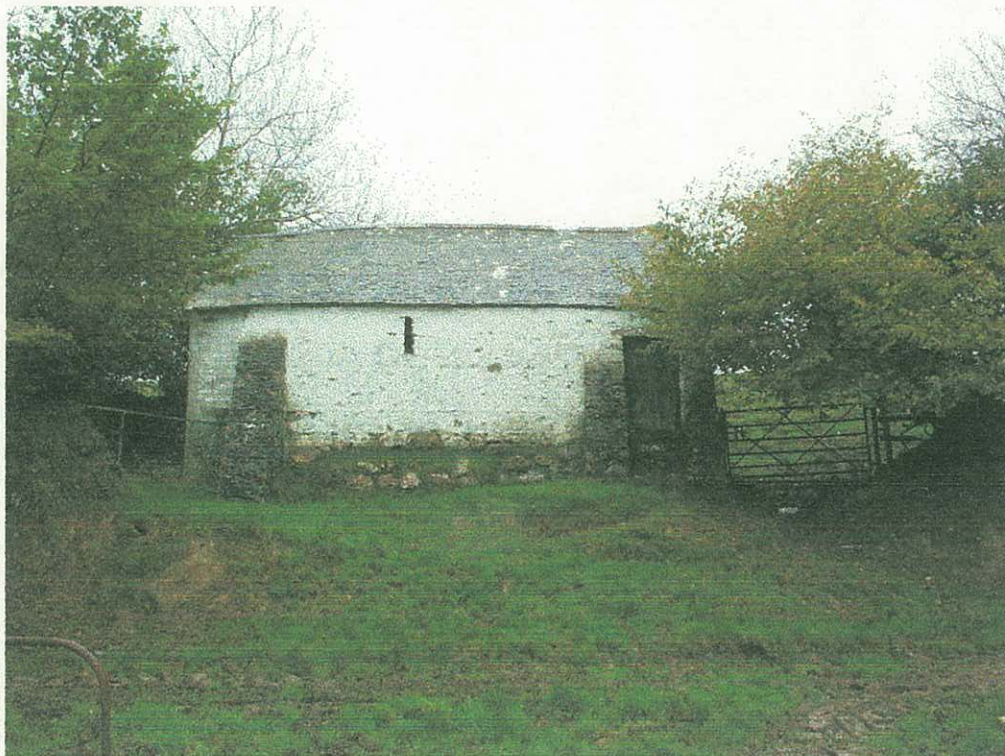
Plate 2: PRN 43770 - 18 th century cartshed. The uneven roofline is caused by severe movement within the roof structure.
