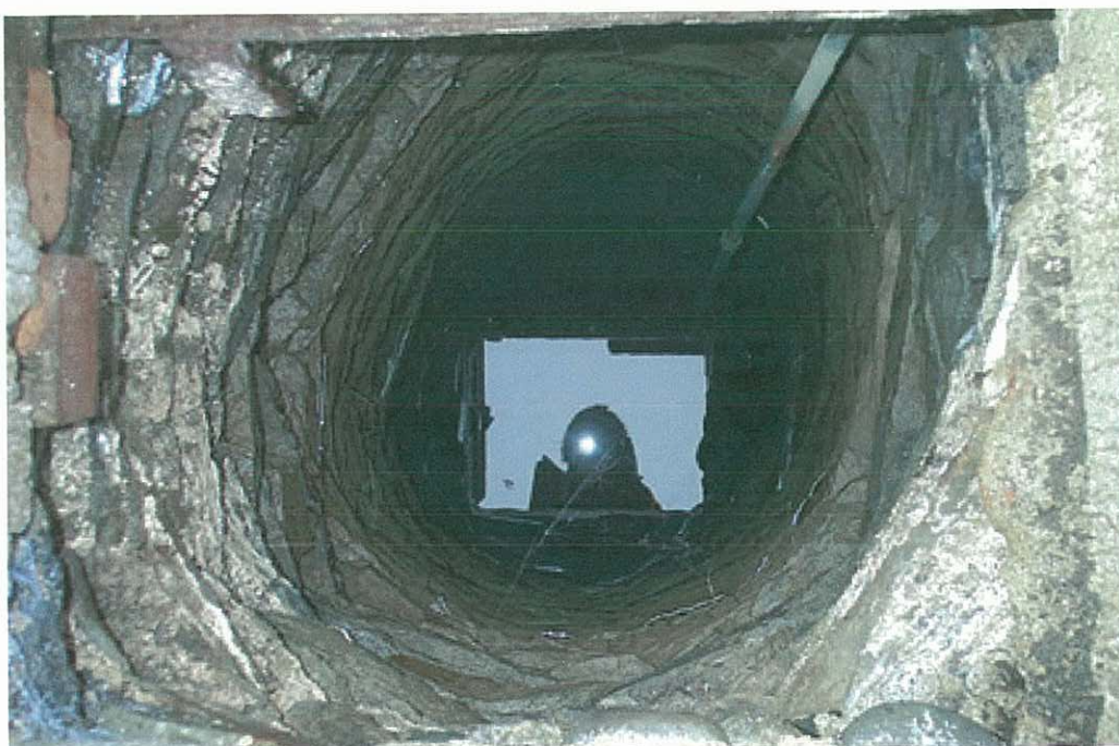
Plate 7 - rubble lined well (PRN42364) to the south of the farmhouse, showing the typical form of the many wells on the farm.
