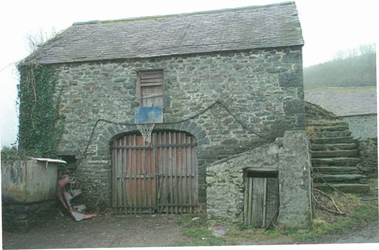
Plate 3 - cart shed (PRN42353) showing poor roof repair and overgrown southern wall
