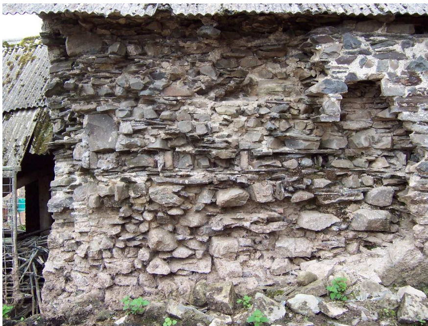
Plate 3 – the exposed wall core on the north elevation, showing blocked ventilation slit (right of centre at base of the wall), also sockets for the first floor joists.
