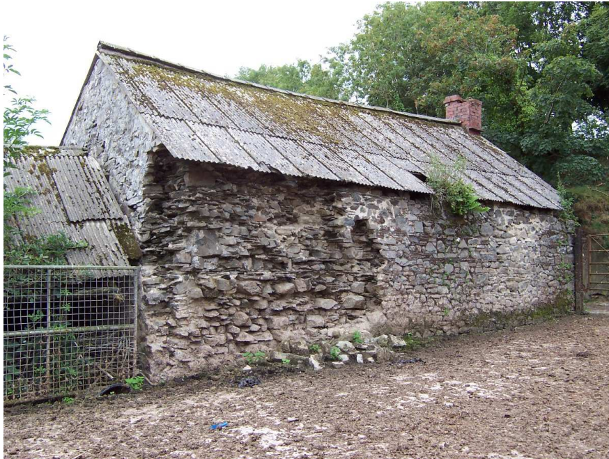
Plate 2 – the north elevation, showing loss of facing stone at the eastern end.
