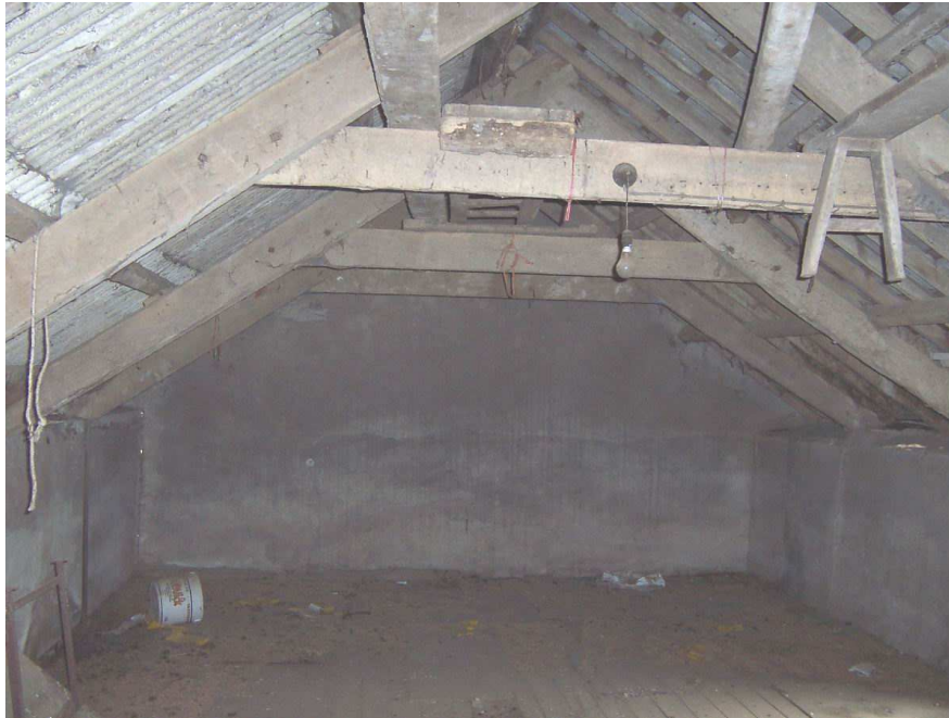
Plate 5 – the interior of the first floor showing the roof trusses
