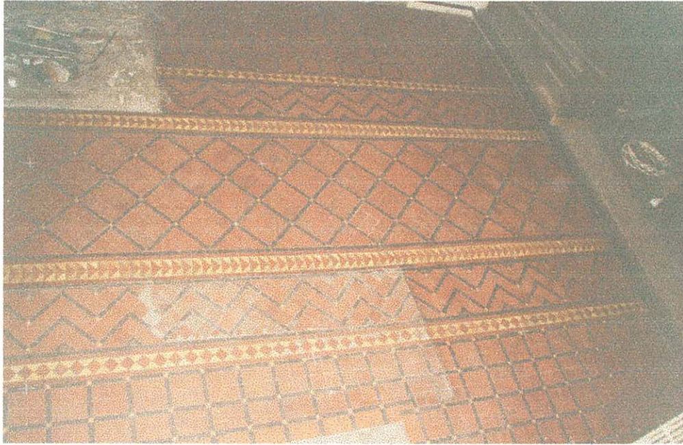
Plate 1: Tiled floor in the chancel prior to removal. The floor was laid in 1876.
