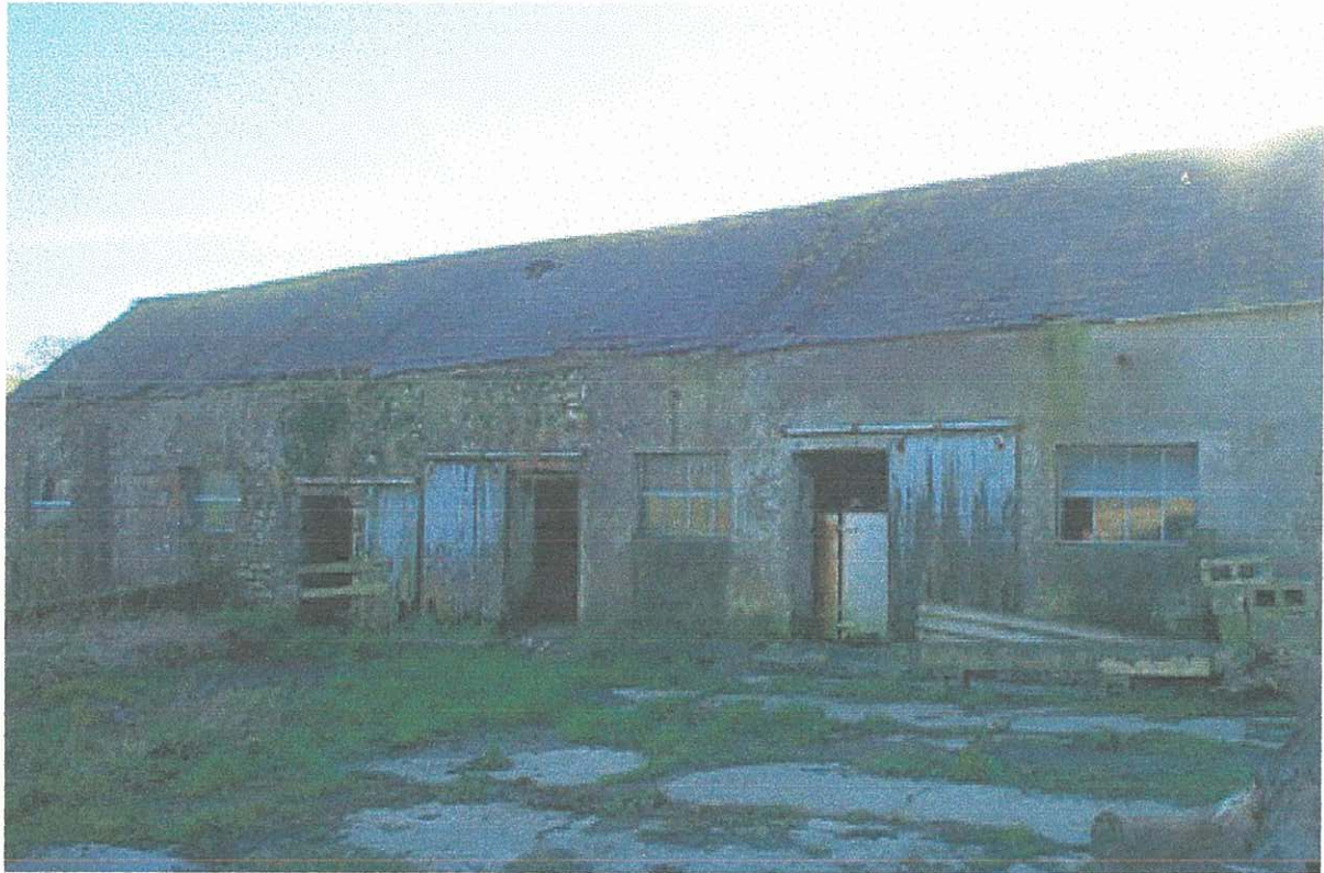
Plate 7 - the cow house from the northeast, showing the poor roof repair and modified exterior and openings.
