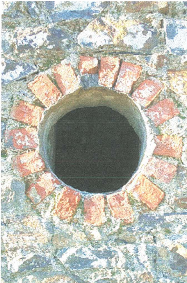
Plate 4 - ventilation oculus with brick surround on the stable block.
