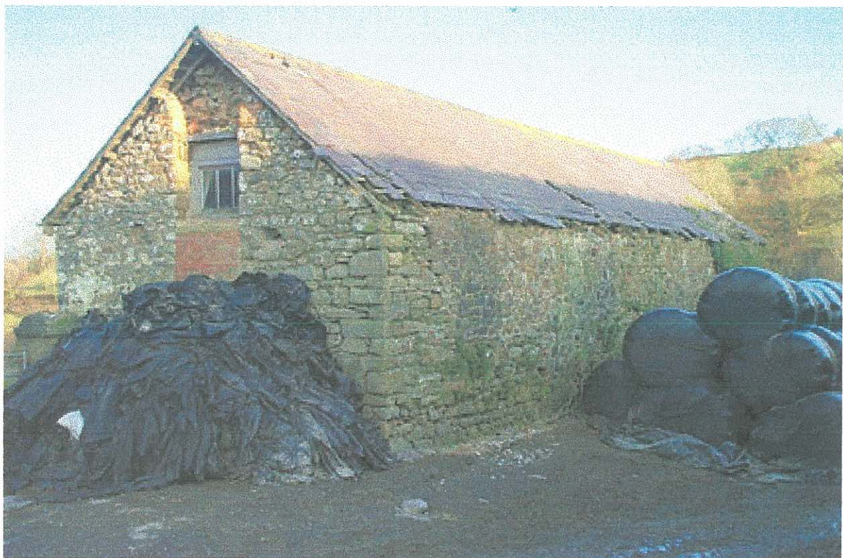
Plate 8 - cowhouse from the southeast showing poor roof repair, overgrown walls and modified openings.
