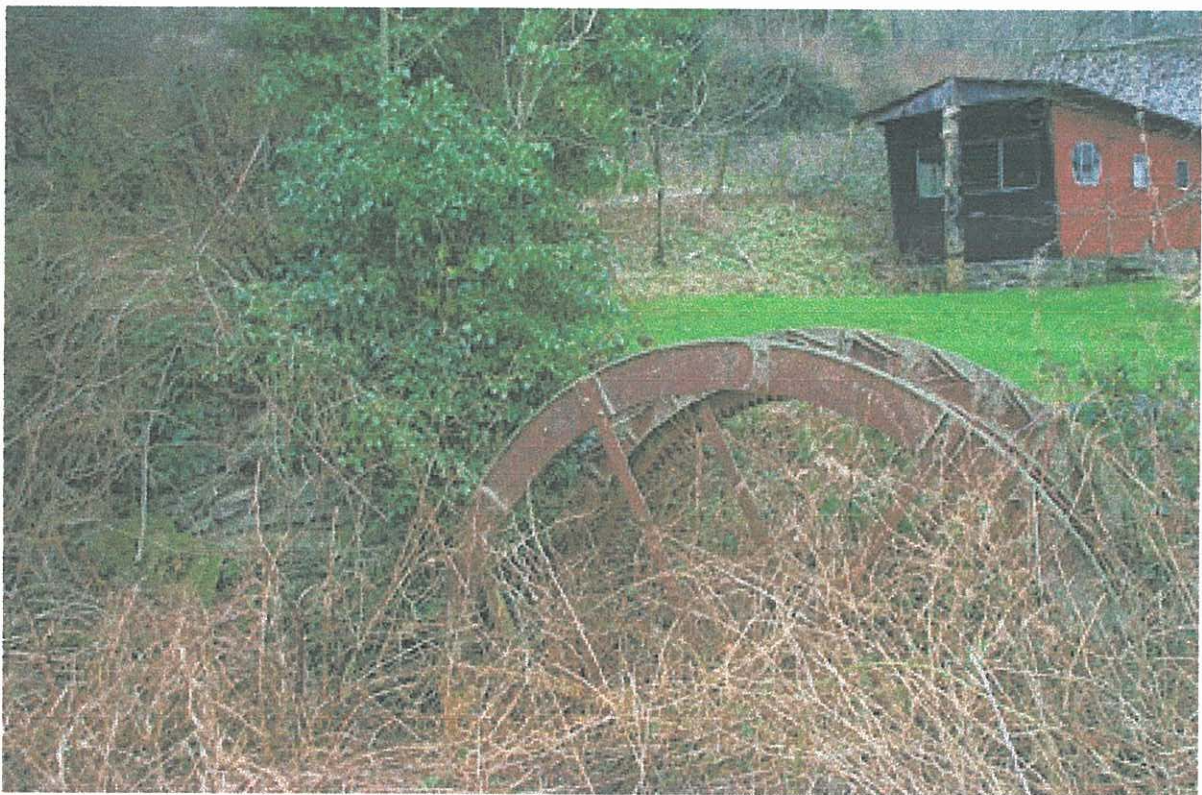
Plate 4 - the overgrown overshoot waterwheel and wheelpit.
