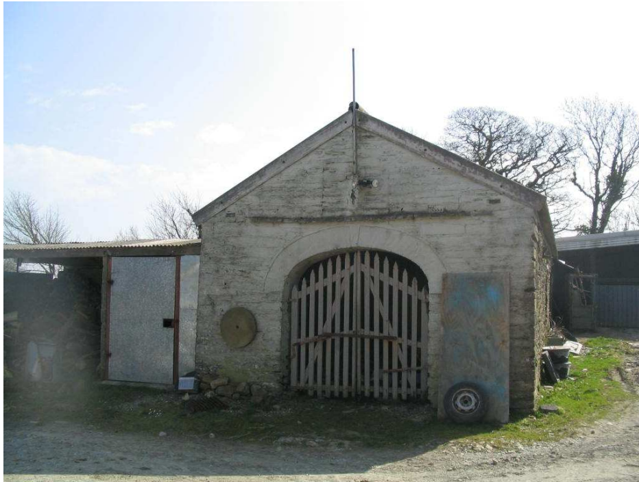
Plate 1 (above) The cart entrance in the northwest gable. Note the dressed stone archway and the projecting slate course above it. These appear to be a kind of architectural 'signature' of Glynhenllan Uchaf.
