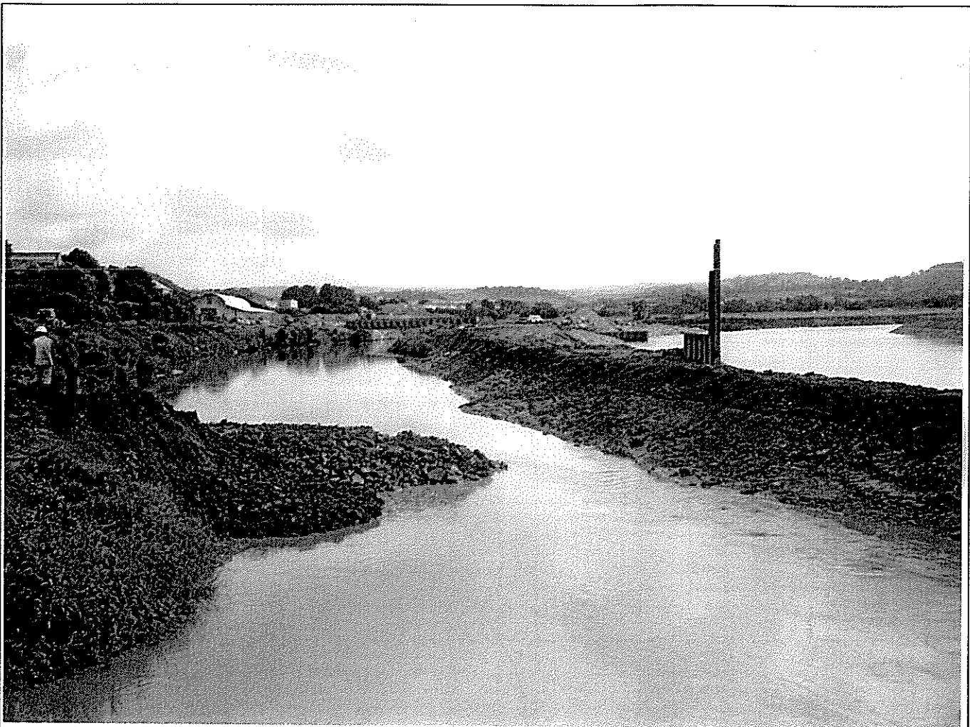
Plate 1: Draining the Afon Tywi during river diversion works. The new channel is to the right.
