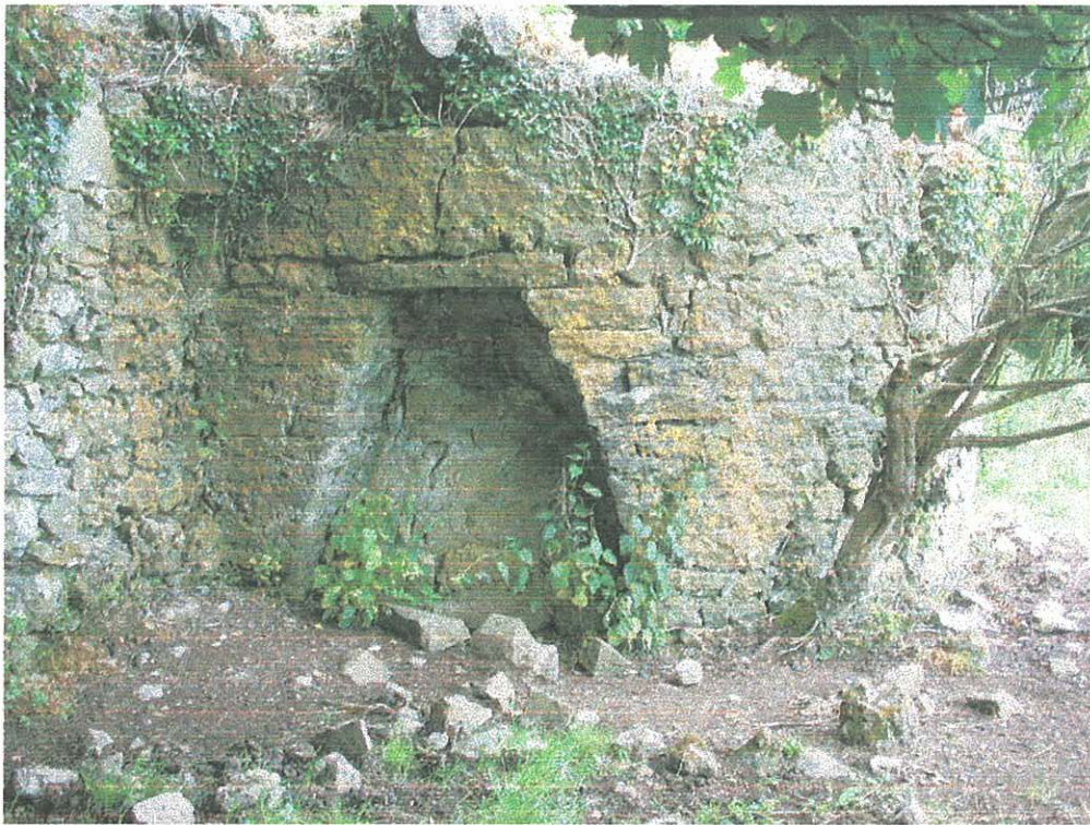
Plate 1 – the lime kiln (17340) showing the drawing arch and overgrown superstructure.
