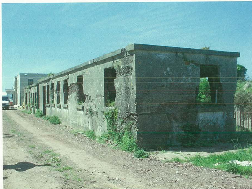
Plate 2 – Chapel Bay Fort (PRN 7655), this building is an early example of unreinforced concrete construction.
