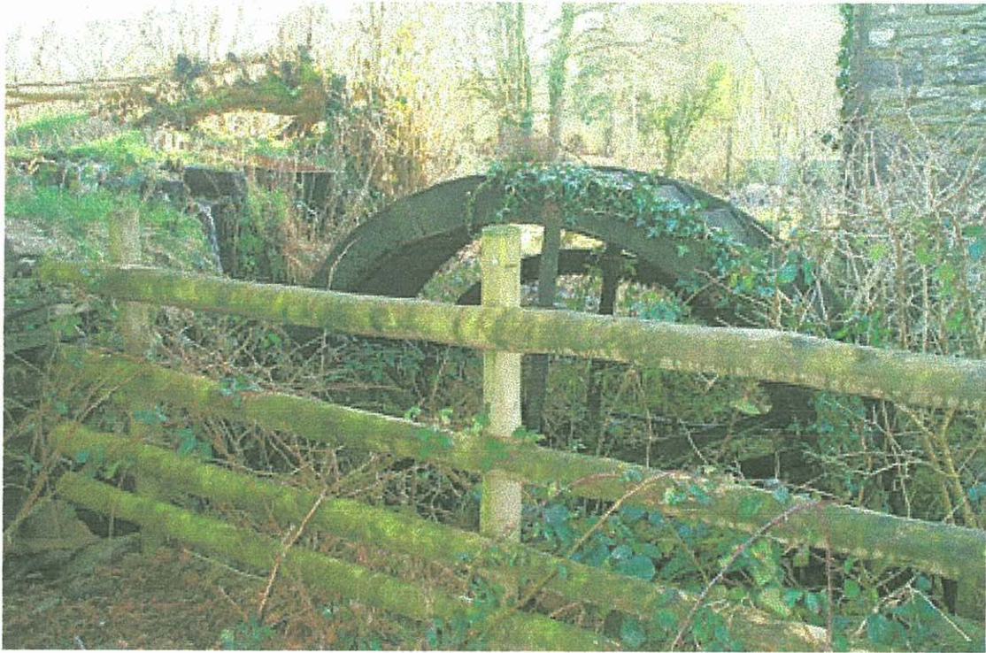
Plate 9 - the overshot water wheel and overgrown wheel pit.
