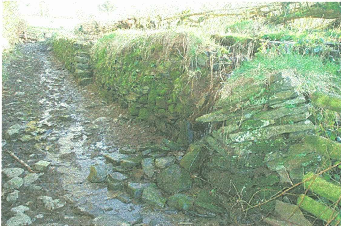
Plate 7 - the drystone wall alongside the raised head race, showing the recently repaired section to the left and the section in need of repair to the right.
