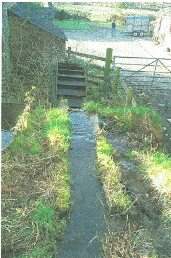
Plate 8 - the wooden launder immediately to the east of the mill wheel.
