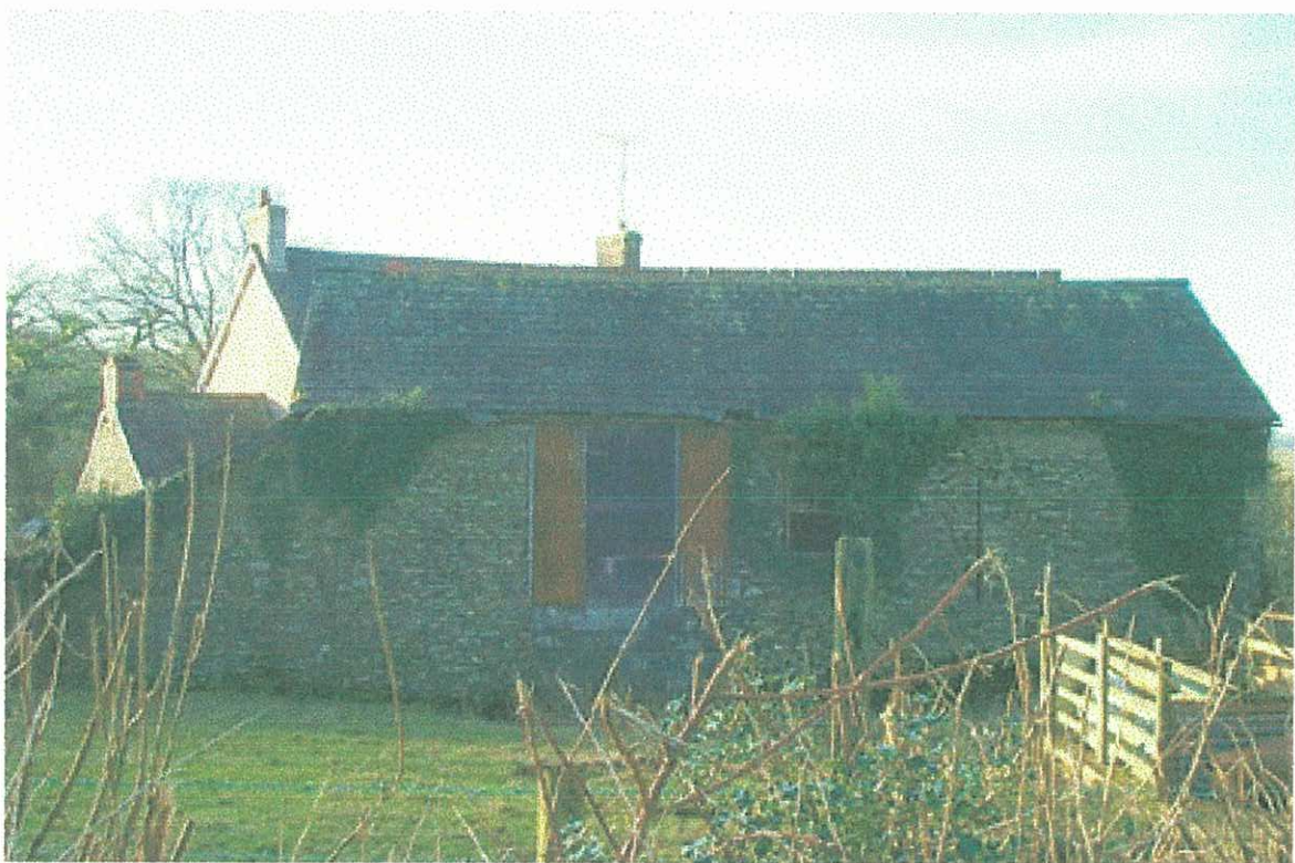
Plate 2 - the threshing barn from the east showing the blocked in entrance, ivy growth and poor roof condition.
