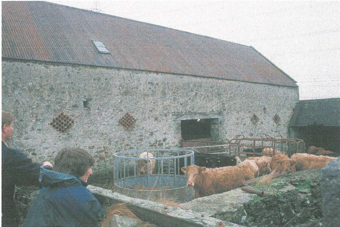
Plate 3: PRN 39364 - large barn at Brownslate Farm. Note the geometric pierced brick ventilation holes.
