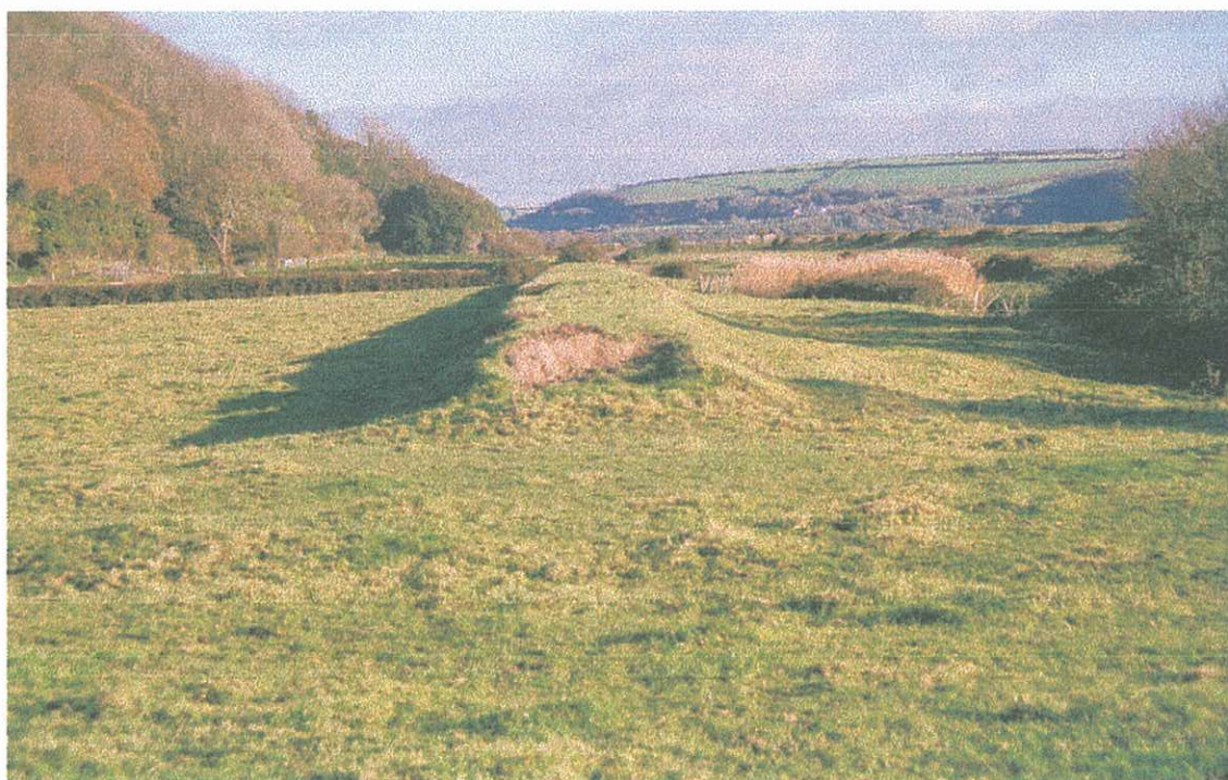
Ground Photograph of sea wall 39291, showing earth construction.
