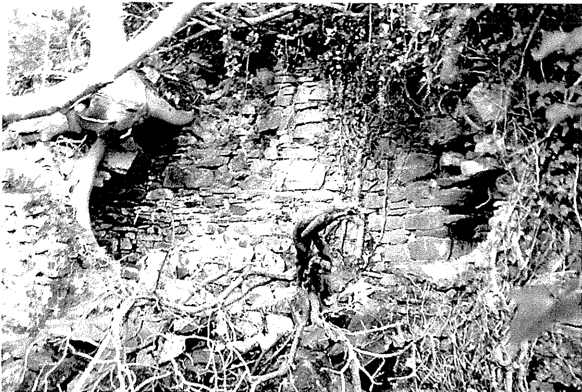
Fig. 2; "Double oven" in eastern wall of westernmost room at Penycwm Slack farm. The oven recesses appear to have been either side of an inglenook fireplace, which has now collapsed and is only represented by the rubble heap in the foreground.
