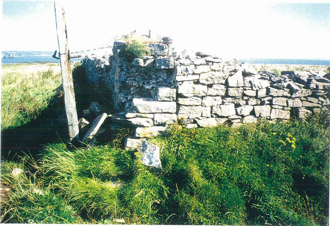
Decayed end of wall and junction (butt joint) between two phases of field walls - west end Caldey Island..
