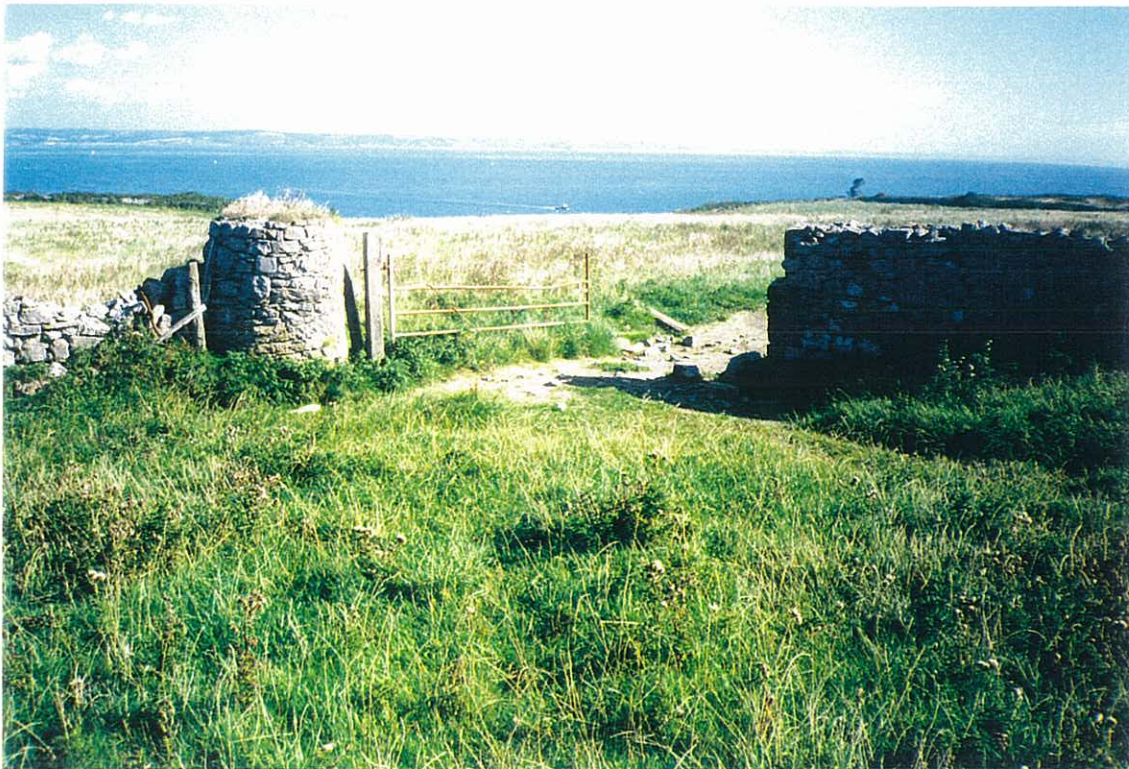
Characteristic semi-circular gate pier on one side of entrance and a wall cut back and pier removed for a modern (now decayed) gate - west end Caldey Island
