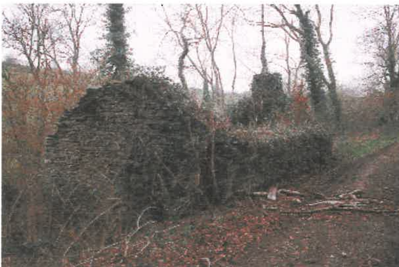
Plate 12: Cwrt-y-gamil (PRN 37858) is an example of what would, in the experience of the 1999-2000 DRS project, qualify as a relatively well preserved cottage. Although roofless, ivy-covered and decaying, the structure still stand to original gable and wallplate height and features such as fireplaces, entrances and windows can be identified. Vegetation obscures the surrounding area, but it is apparent that a garden plot also exists.
