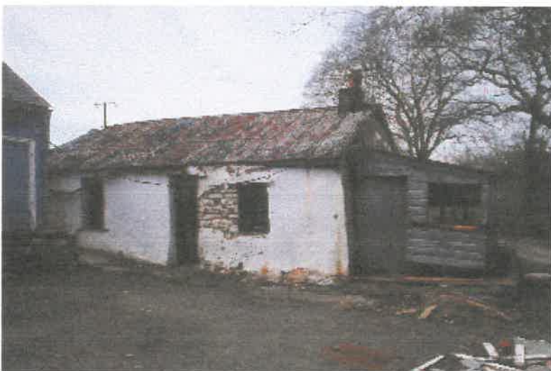
Plate 15: This cottage in southern Ceredigion will remain anonymous in this report as it is subject to a planning application which will involve demolishing the building to make way for a new dwelling. It is part clom-built and the need to record and/or preserve the diminishing examples of this type of structure is becoming increasingly important as their number dwindles.
