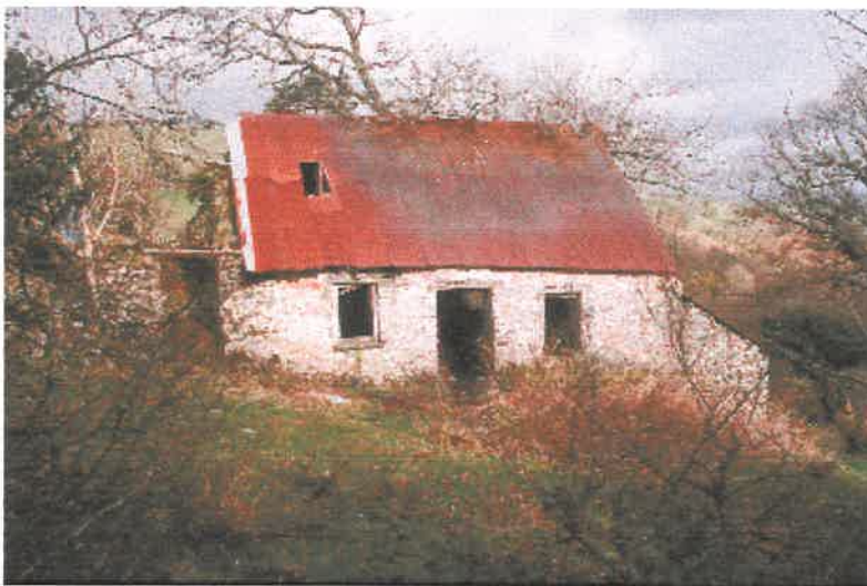
Plate 17: A well preserved cottage at Bryn Pribwll, Llansadwrn. Although outwardly in apparently good condition, this stone built structure's earth bonded fabric is beginning to collapse at the rear and it is unlikely that the structure will survive many more winters unless major repairs are undertaken. The likelihood of that happening in the case of a great number of rural cottages of this type is of course very small.
