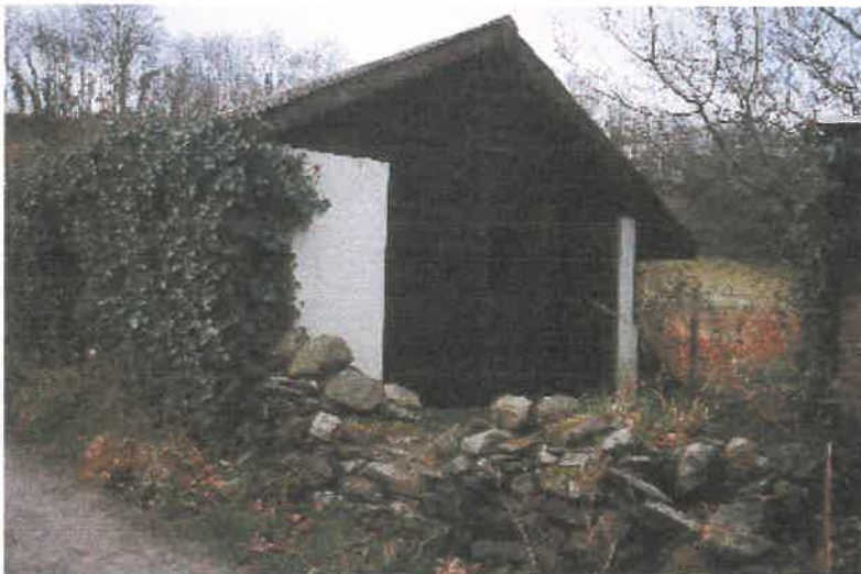
Plate 14: PRN 37809, Penybanc Bach, is an example of a 19th century cottage which has been, in part, salvaged for an alternative use. Half of the building has been incorporated into a modern shed; the other half probably robbed of some stone and therefore now only defined by low wall bases.
