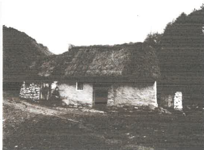
Plate 2: Thatched cottage in the Llandovery area, late 19th century. This demonstrates how small many rural cottages were, and also how they were often extended by the addition of lean-tos. If reduced to wall bases, the plan of a cottage such as this would probably lead an archaeological fieldworker to record the site as a longhut. The additional cells created by the extensions at either end of the dwelling are often seen in longhuts in both upland and lowland contexts.
