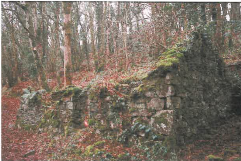
Plate 13: Another 'relatively' well preserved structure (PRN 37848) was described as being associated with a 'grinding mill' on the parish tithe map. The nature of this mill was not established, but the surviving building appears to have been a simple cottage with a central doorway, two windows in the front lateral wall and a small extension built on to the furthest gable wall. The use of fairly large stone blocks in the wall fabric is not typical of the cottage sites visited in the area.
