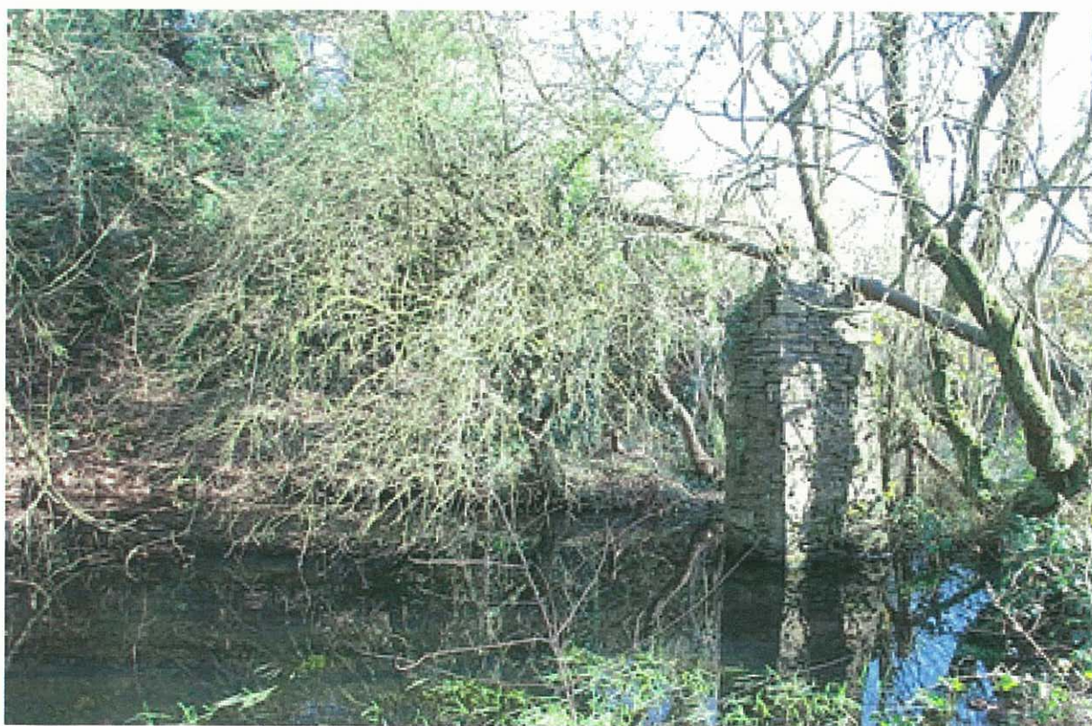
Plate 6 - rubble pillar supporting the pipeline (PRN42307) from the reservoir (PRN42310).
