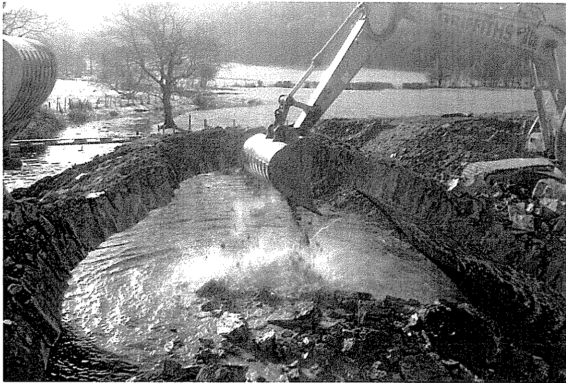
Plate Five: Demolition of the arch of Pontarsais Bridge
