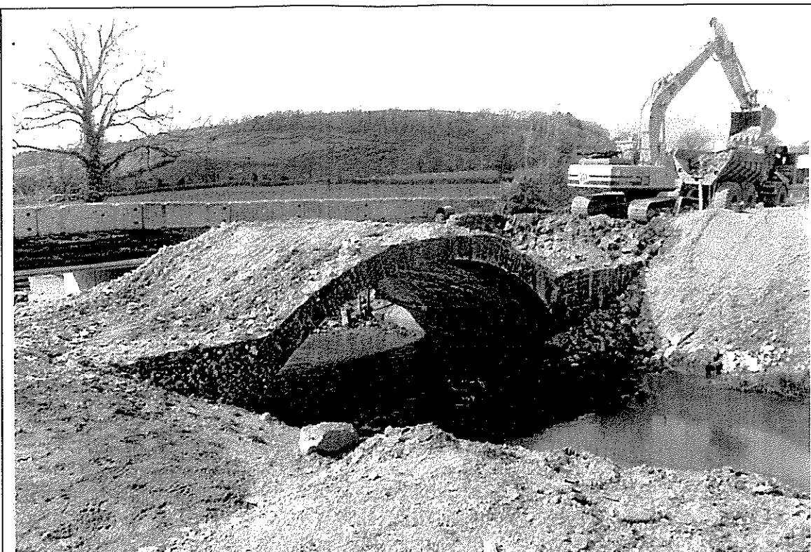
Plate Three: Brick arch structure of Pontarsais Bridge during demolition
