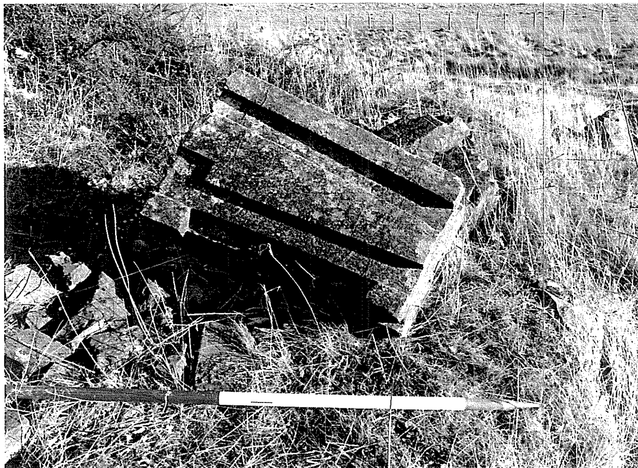
Figure 32: Example of dressed Bath stone from Thomas Johnes' house (PRN 7199)
