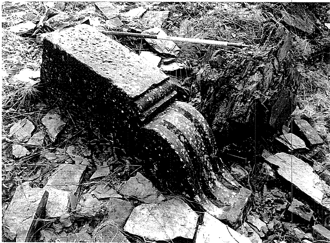
Figure 36: Example of dressed Bath stone from Thomas Johnes' house (PRN 7199)
