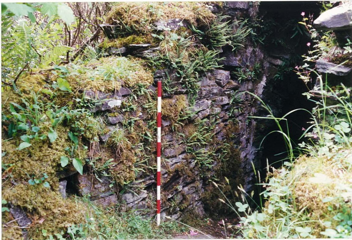
Photo 5. South passageway wall.
