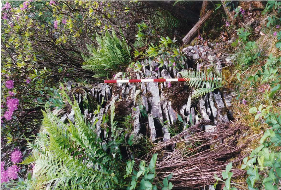
Photo 3. External wall on south-west side.
