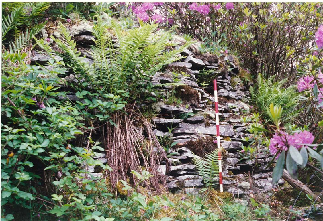
Photo 4. External wall on south side.
