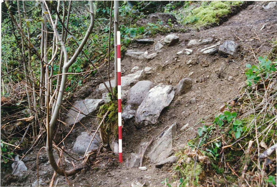
13. Trench 3 showing collapsed revetment.
