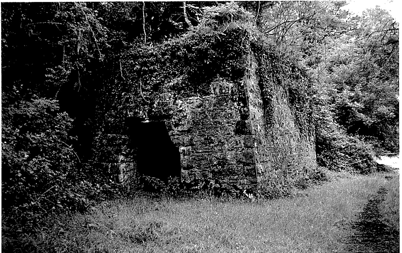
Photograph 29. (Map 15) One of the best preserved and largest of the limekilns in the survey area (34612). Square kilns such as this example are particular to the Pembroke River. The norm on Milford Haven is for round or D-shaped kilns.
