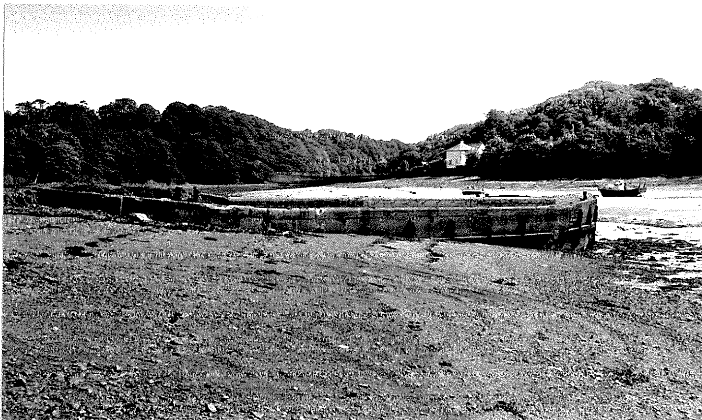
Photograph 10. (Map 6) A pier (34957) constructed from a concrete-filled wreck in Castle Pill, Milford Haven.
