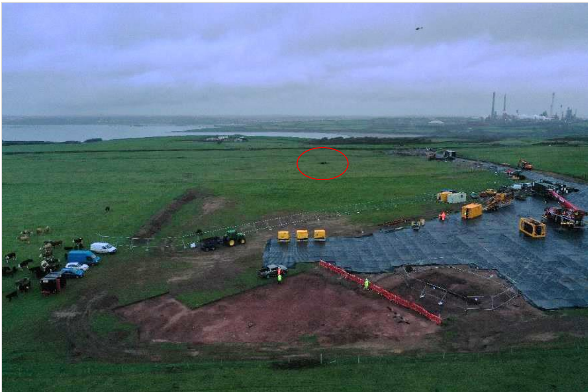
Photo 3: View of groundworks at the Devil's Quoit Area. The haul road and cable trench can be seen running along the right side of the photo, the Devil's Quoit is highlighted in red in the centre and the drilling compound is in the foreground.
