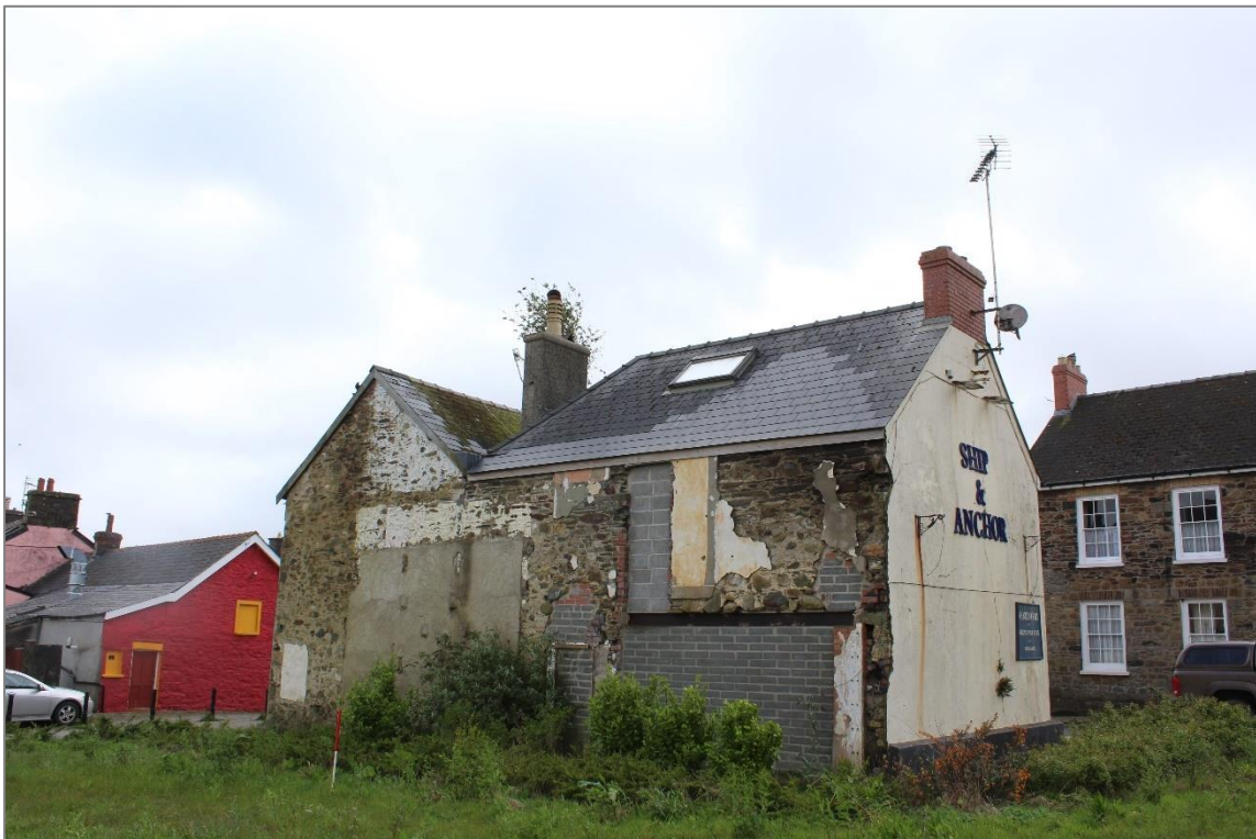
Photo 7: View southeast of the north face of the building. Note extent of modification to the northern edge of the building after demolition of former public library and Victorian wing/function hall. 1m scale.
