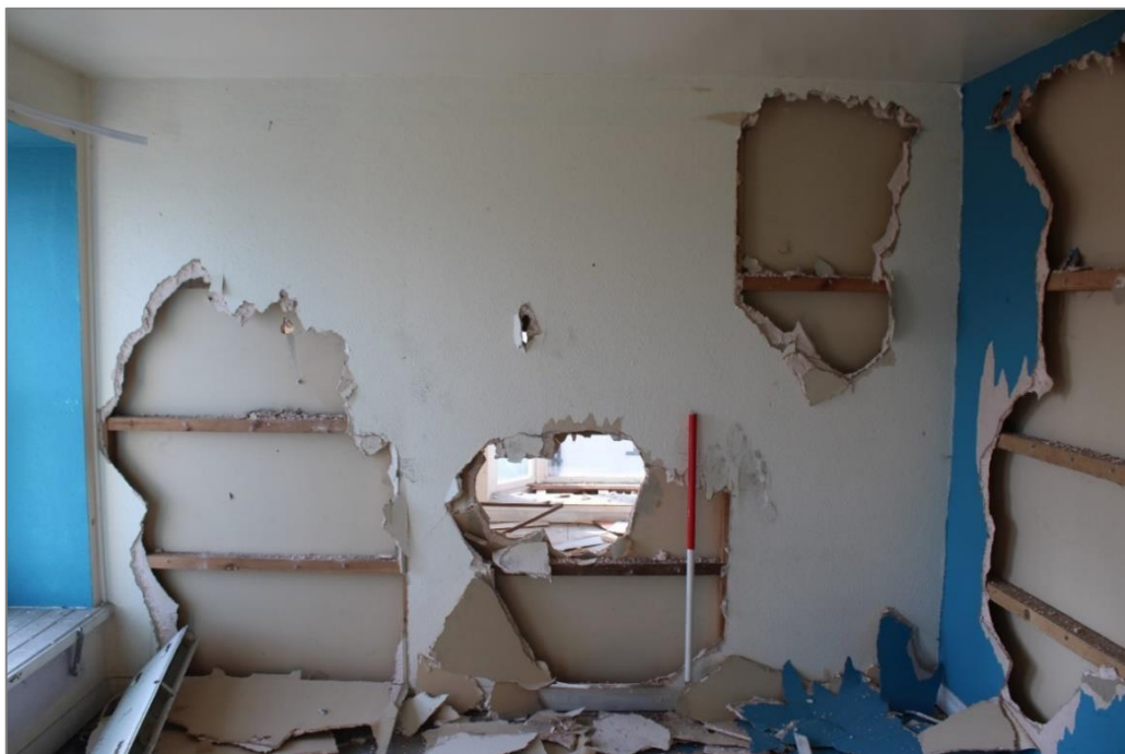
Photo 33: Looking south in room 103. Note plasterboard walls. 1m scale.
