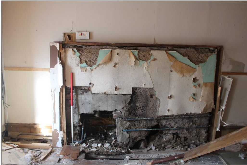
Photo 28: Looking at former fireplace with remains of back boiler on western wall of room 102. Looking west, 1m scale.
