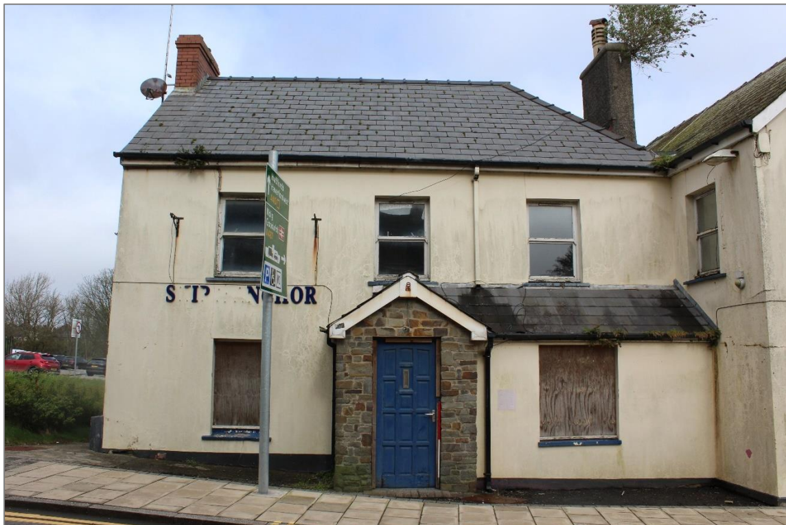
Photo 3: View north of the front (south) face of the western block. 1m scale. Note modern porch and extension to the right.
