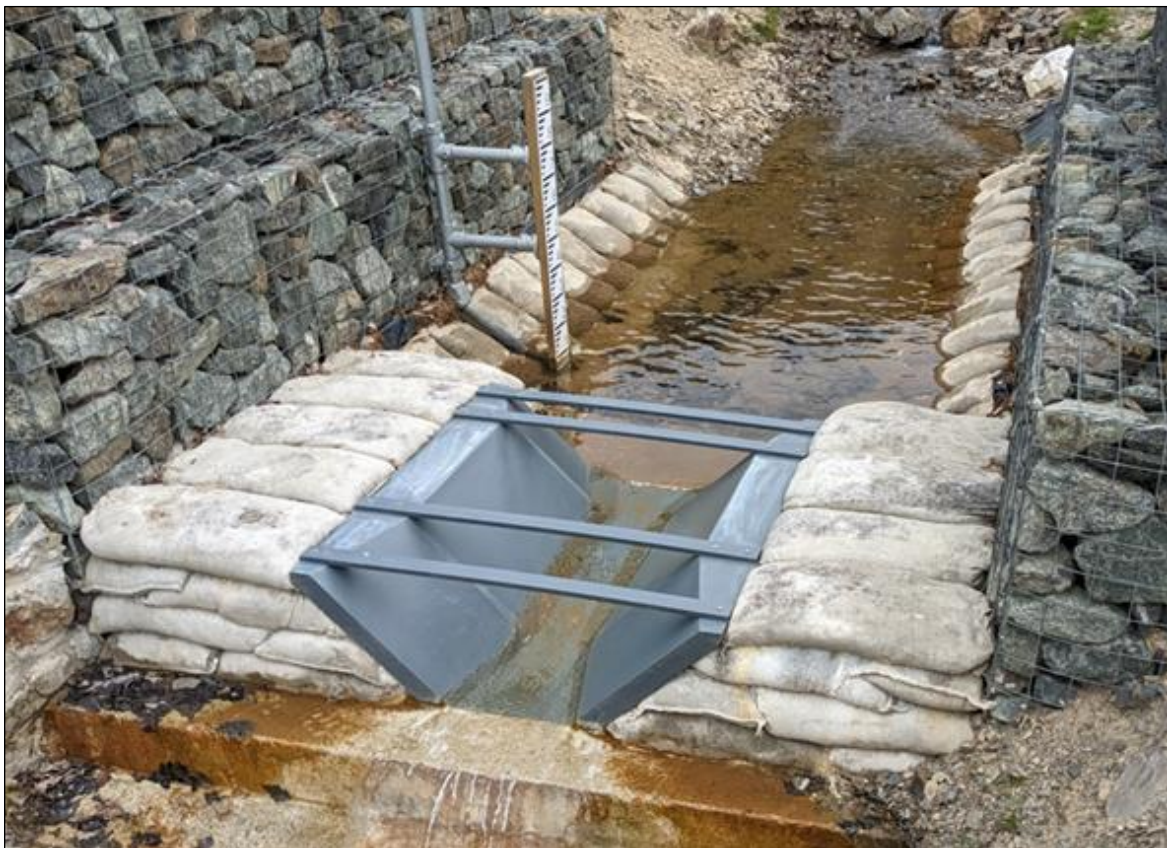
Figure 10: Example of the flume to be used in the flow monitoring structure.
