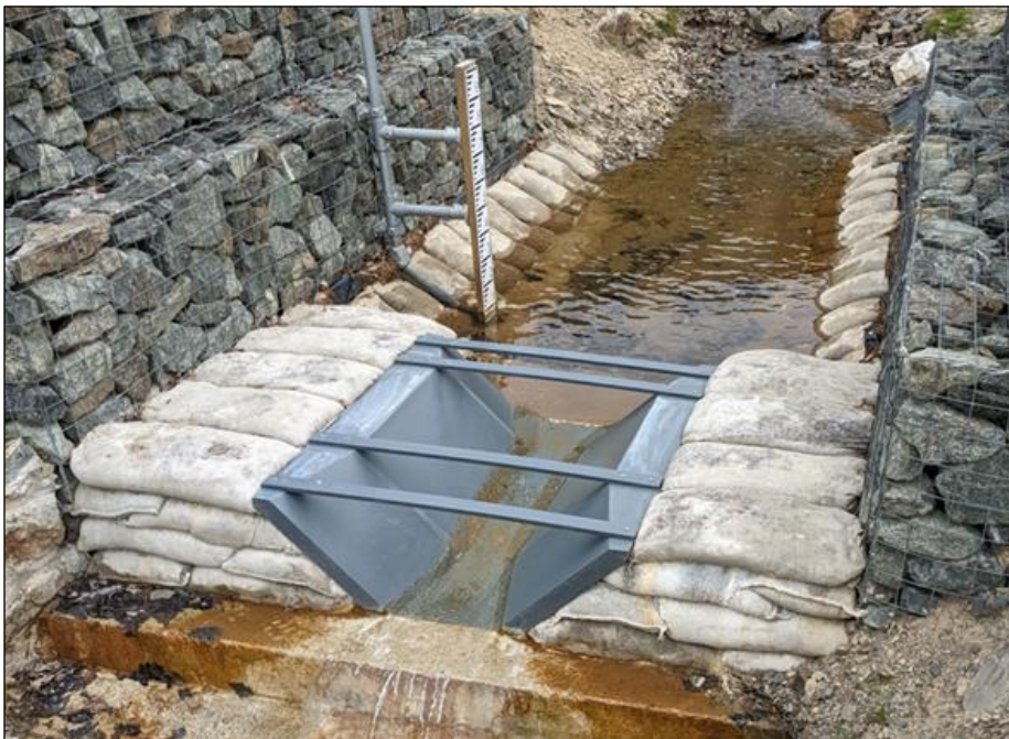
Figure 12: Example of the flume to be used in the flow monitoring structure.
