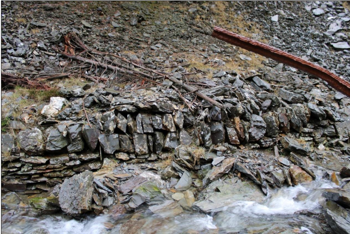
Photo 23: View west of wall PRN 36761, showing some of the changes from the horizontal masonry on the left to vertical masonry in the centre.
