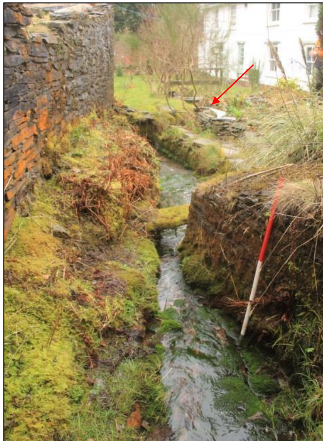
Photo 5: View northwest along the line of water channel as it emerges from Level Fawr adit. On the right the brick built modern culvert intrudes, with the diverted water course heading to the left, the original line lies to the right (arrow). 1m scale.
