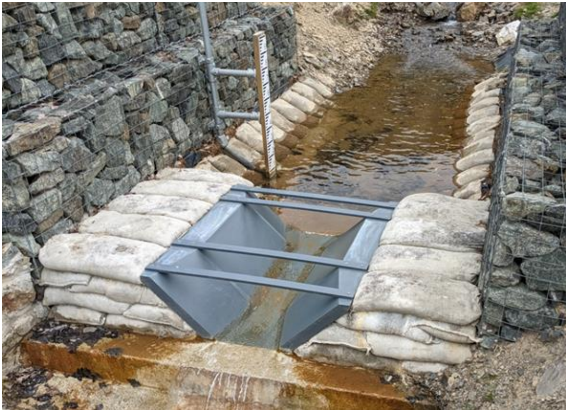
Figure 10: Example of the flume to be used in the flow monitoring structure. The proposed structure will not use a concrete base or stone gabions illustrated in this example.
