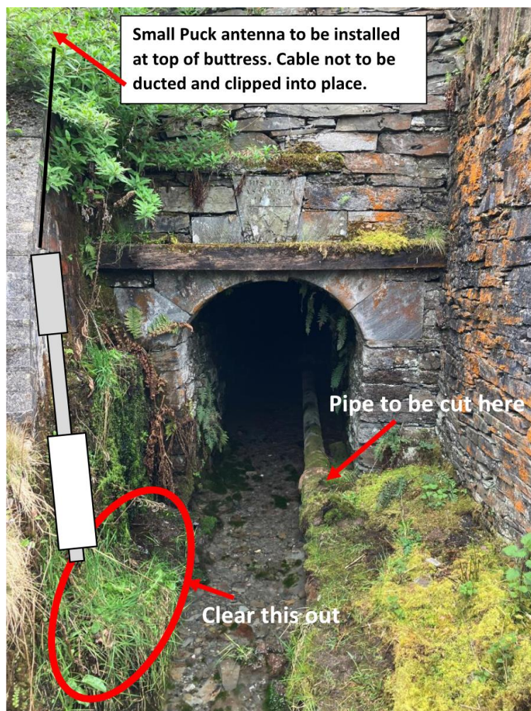
Figure 11: Image demonstrating development proposals and location of data logger and sensor on the left.
