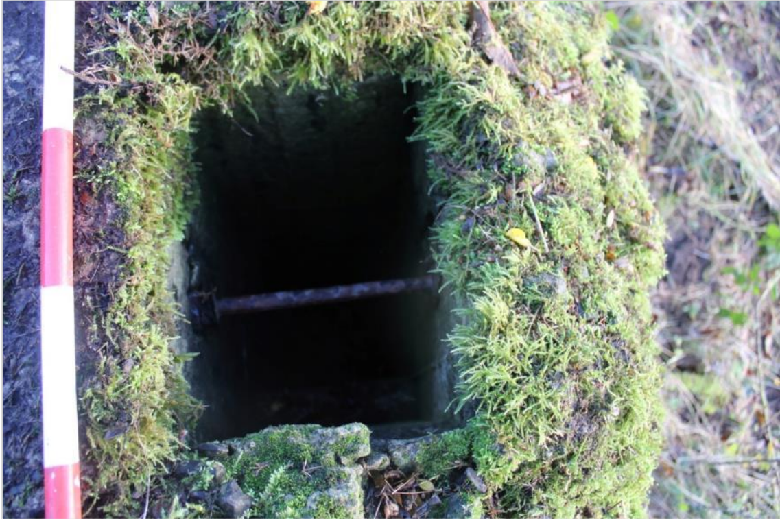
Photo 12: Void in top of concrete block. 1x0.5m scale.
