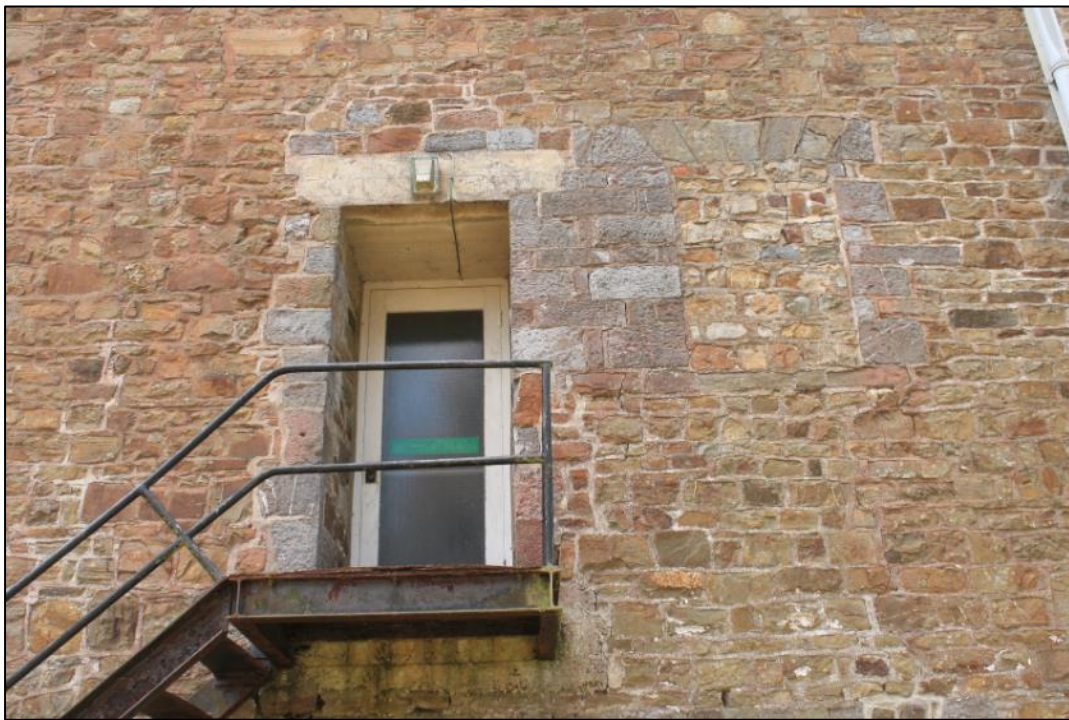
Photo 34: View west showing detail of the first floor openings, with inserted doorway.
