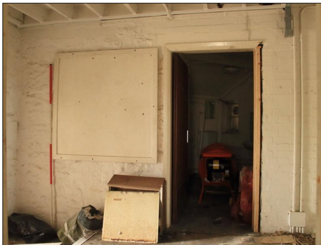
Photo 52: View west, showing the inserted opening and brick surround on the west side of the lobby. 2m scale.
