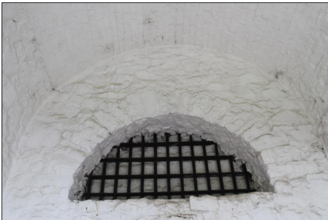
Photo 44: View south, showing the barred light above the doorway, with brick-vaulted ceiling above.
