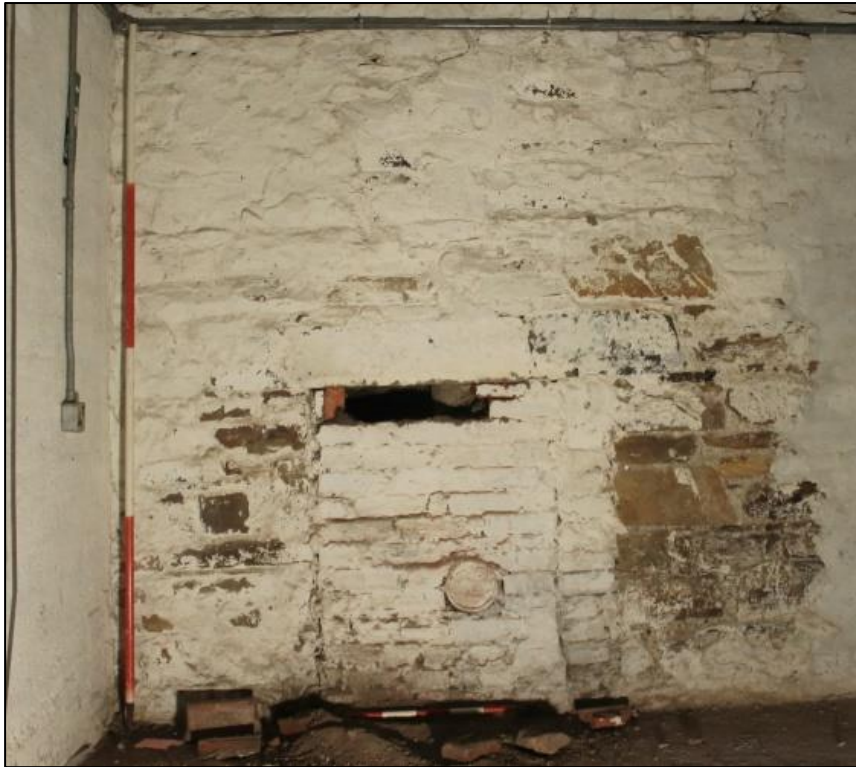
Photo 91: View east, showing detail of the blocked fireplace. 2m and 0.5m scales.
