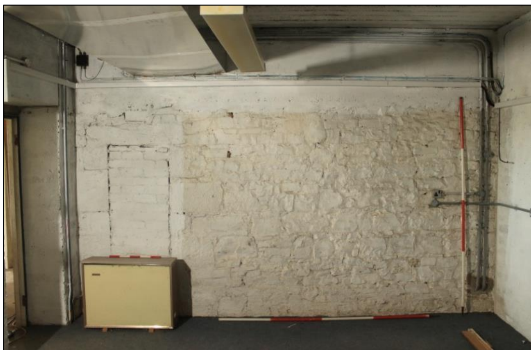
Photo 78: View east, showing the east wall of the small strongroom, with blocked doorway on the left. 2m and 0.5m scales.
