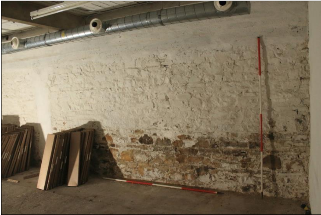
Photo 89: View south from the northernmost of the two rooms, showing the dividing wall between the two western strongrooms with an area of repair covered in plasterwork to the left of the photo. 2m scales.
