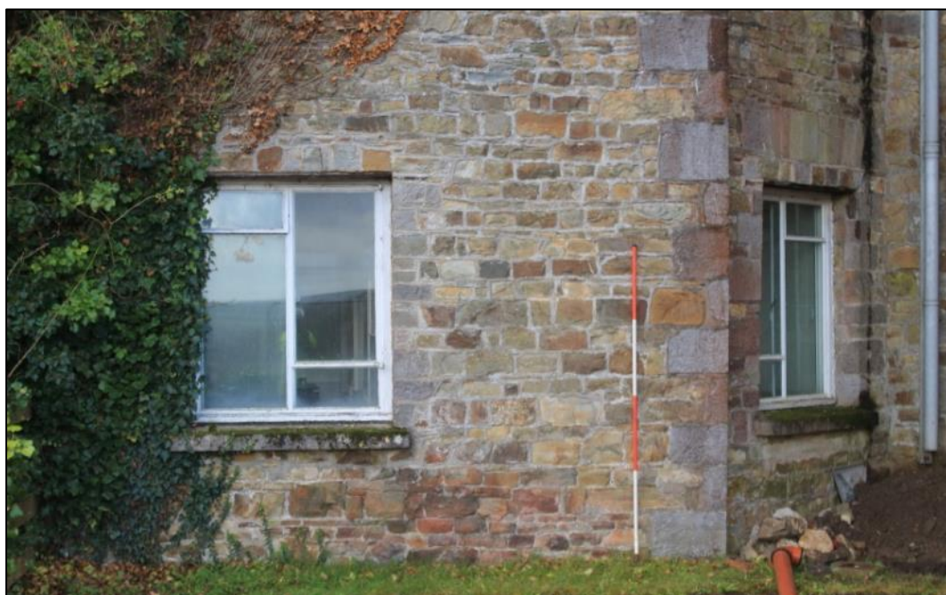
Photo 27: View south, showing the modern windows replacement in the projecting gable at ground floor level. 2m scale.
