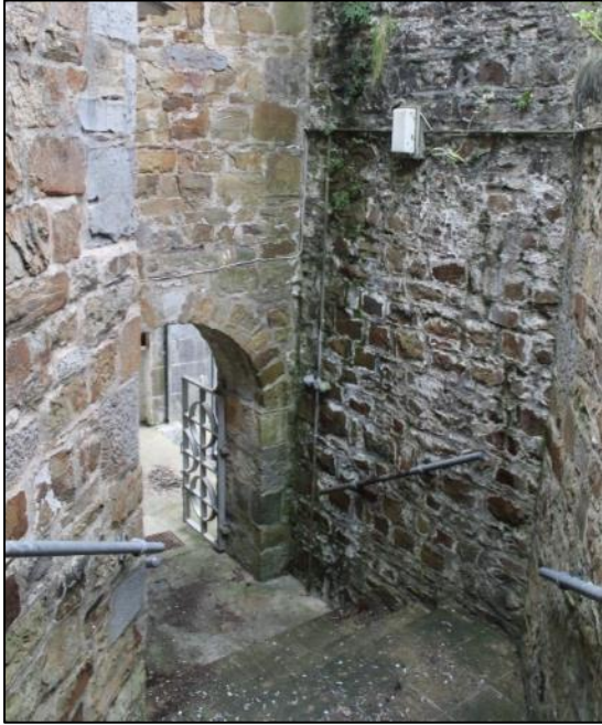
Photo 95: View southeast down the first floor stairway access, with 1960s masonry on the left, 1970s masonry on the right.
