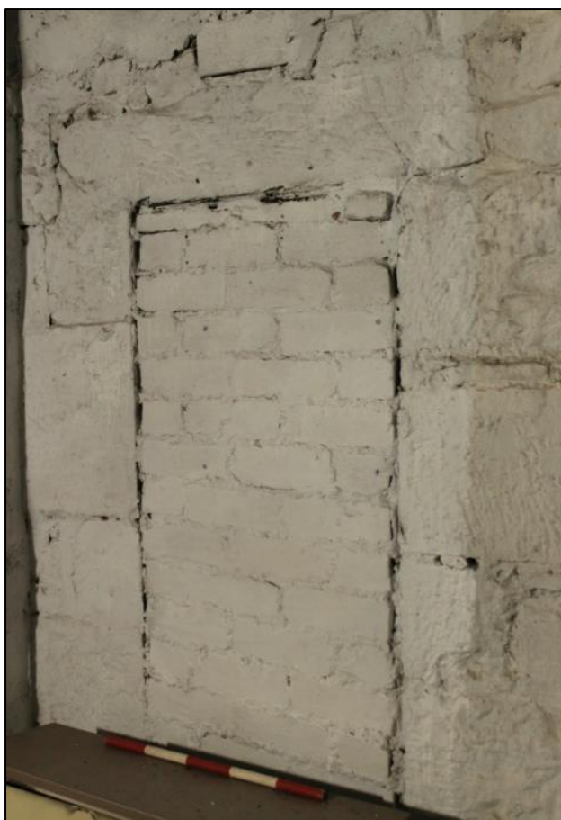
Photo 79: View east, showing detail of the blocked doorway in the east wall of the small strongroom. 0.5m scale.
