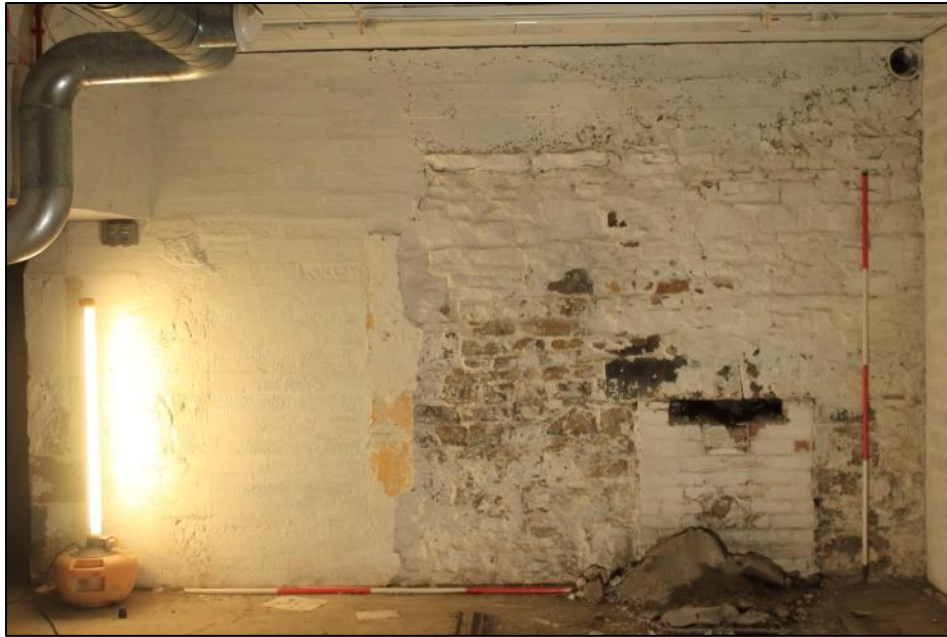
Photo 75: View west, showing the west wall of the northeast strongroom. The blocked fireplace opening is visible on the right and a blocked doorway on the left. 2m scales.
