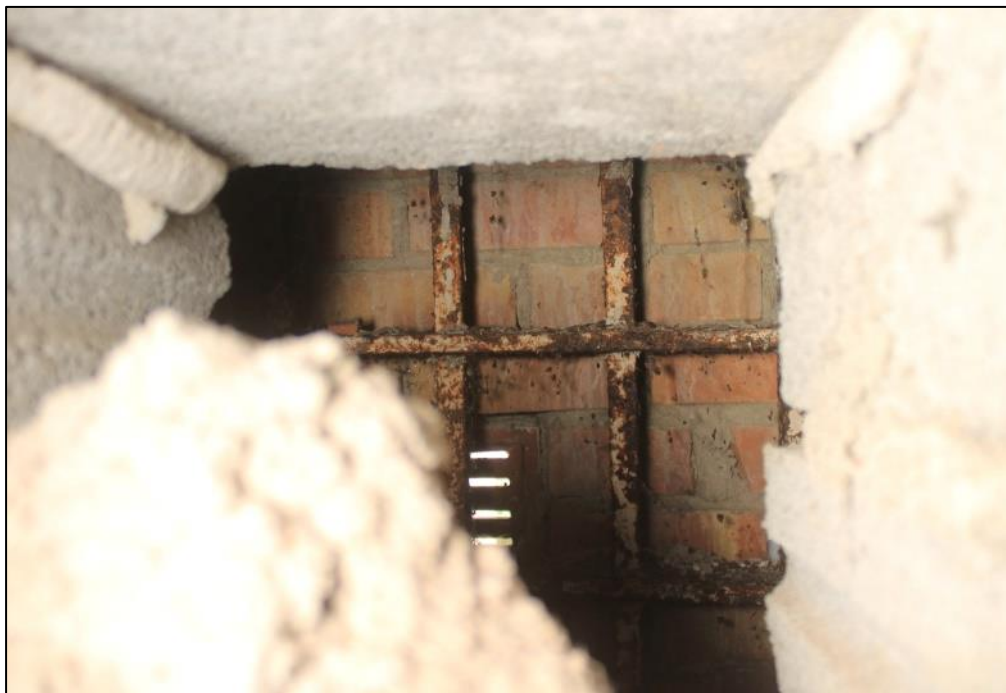
Photo 72: View south, showing the original window bars behind the breezeblock insert.
