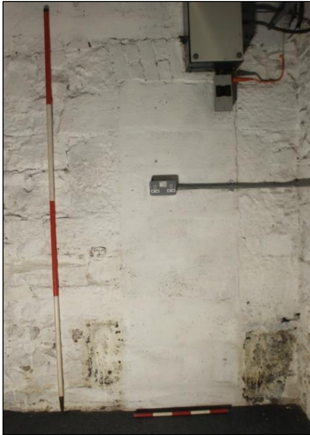
Photo 81: View west, showing detail of the blocked doorway in the west wall of the small strongroom. 2m and 0.5m scales.
