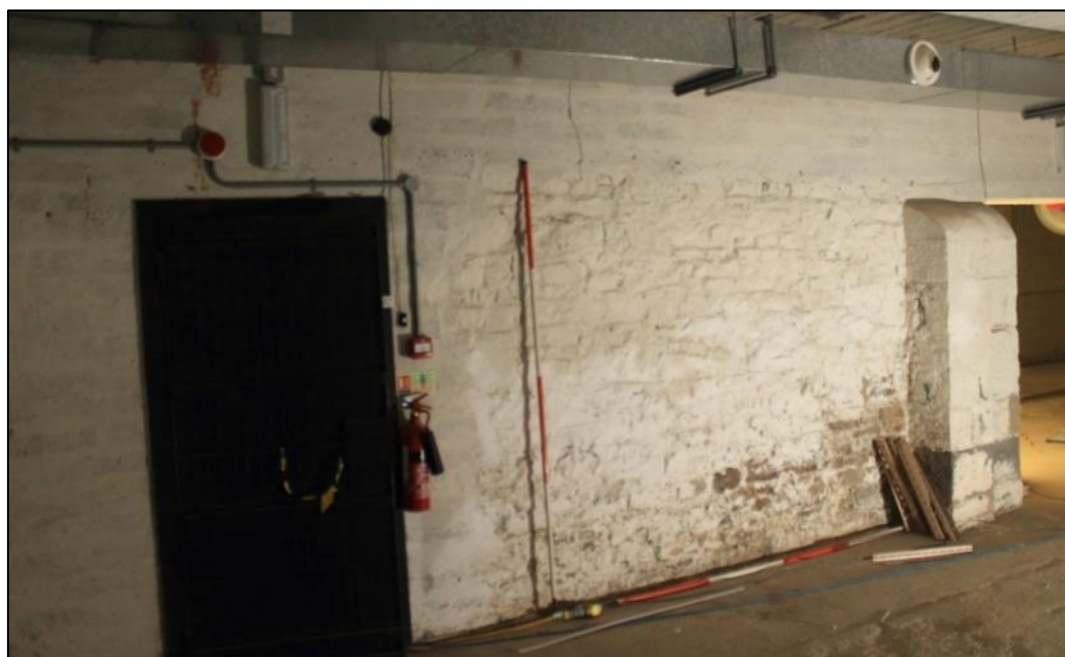
Photo 68: View north, showing the inserted opening on the left and part of an original doorway protruding on the right. 2m scales.
