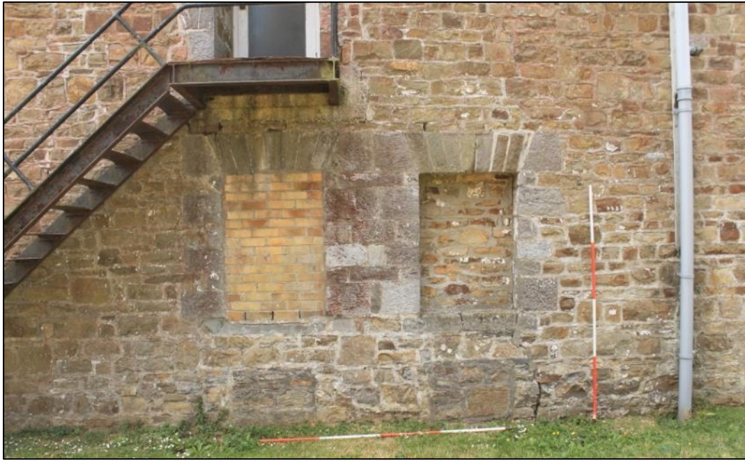
Photo 33: View west showing detail of the blocked ground floor windows with blocked heating vents below. 2m scales.
