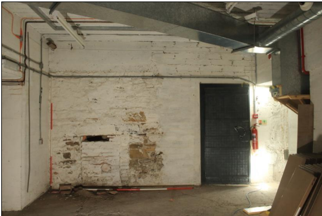
Photo 90: View east, showing the eastern wall of the strongroom, with blocked fireplace on the left and inserted steel door on the right. 2m scales.
