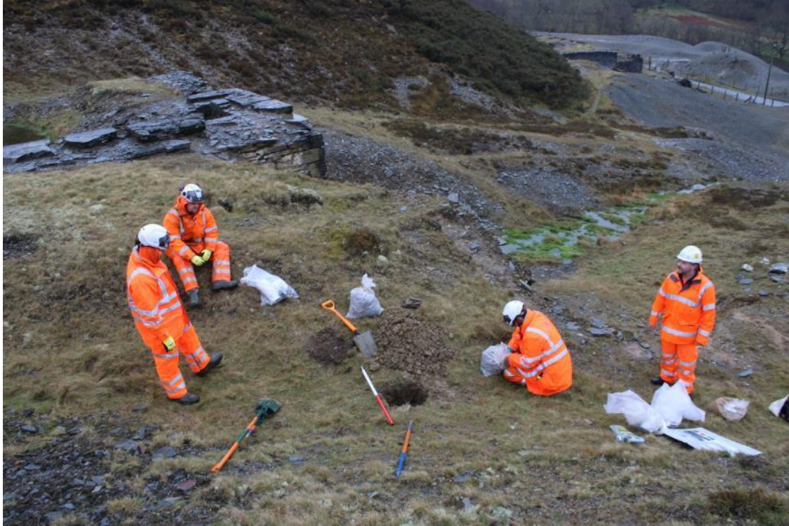
Photograph 2: Hand digging the geotechnical test pits in 2023.
