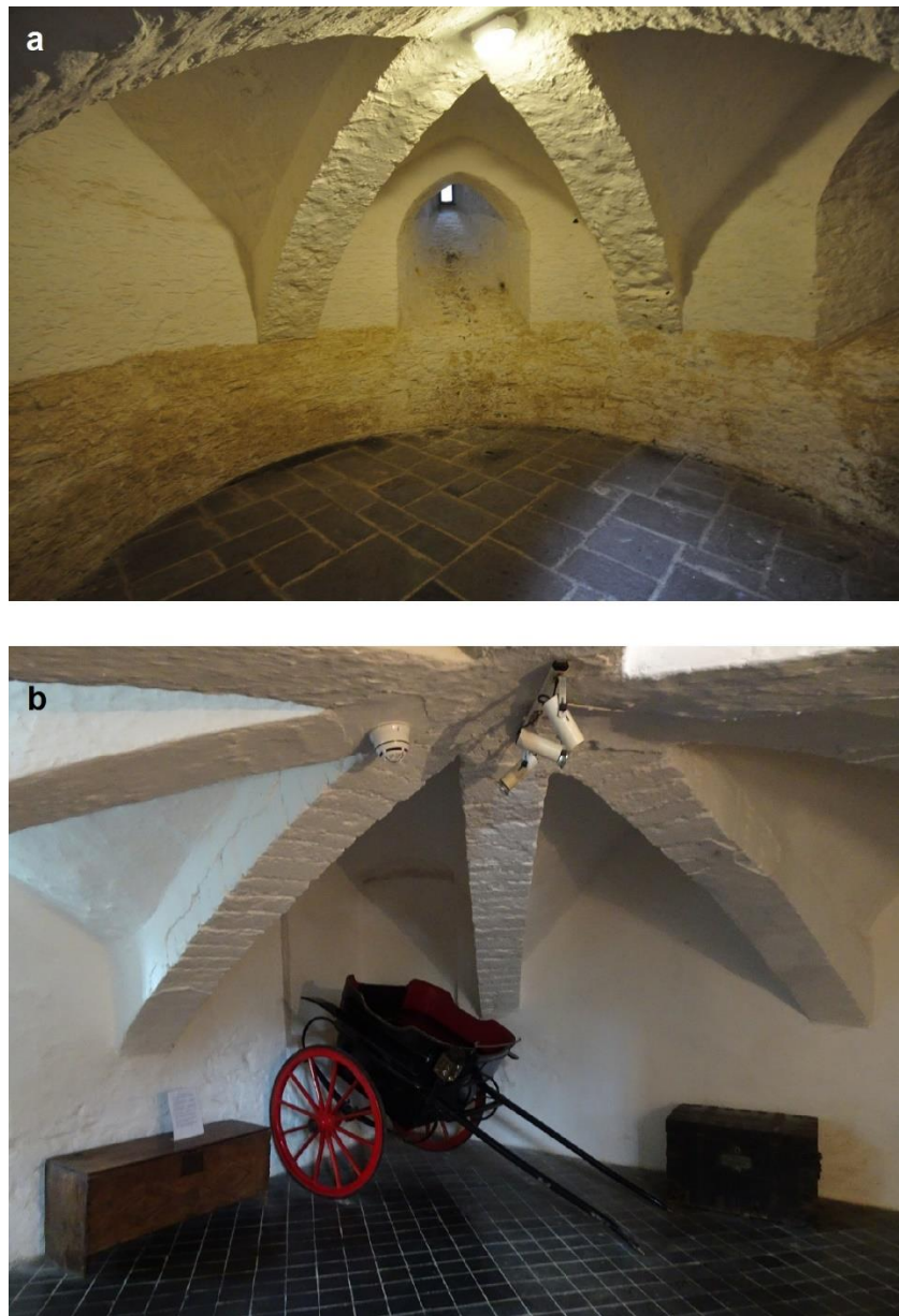
Fig. 196: Low rib-vaults with a deep extrados at a) Castell Coch (Glam.), late 1260s-70s; b) Picton Castle northeast tower
