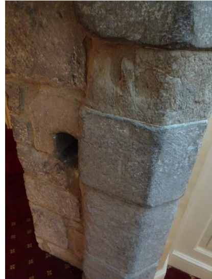
Fig. 132: Medieval doorway S23-4: drawbar-socket in east reveal, looking northeast
