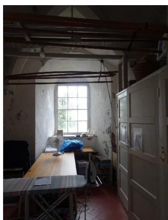
Fig. 76: Southern undercroft central bay G10b, looking south
