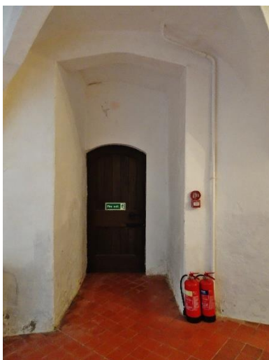
Fig. 72: North wall east opening G9-2, looking north
