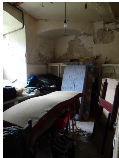
Fig. 79: Northeast corner of Northwest Tower room G11a, showing diagonal squinch
