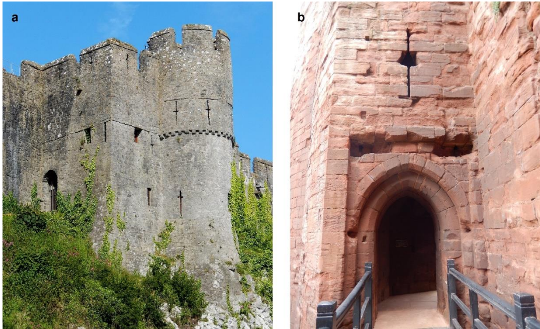
Fig. 195: Cruciform loops in Aymer de Valence's castles at a) Pembroke (St Ann's Bastion); b) Bothwell, Lanarks. (donjon). Both c.1300-10
