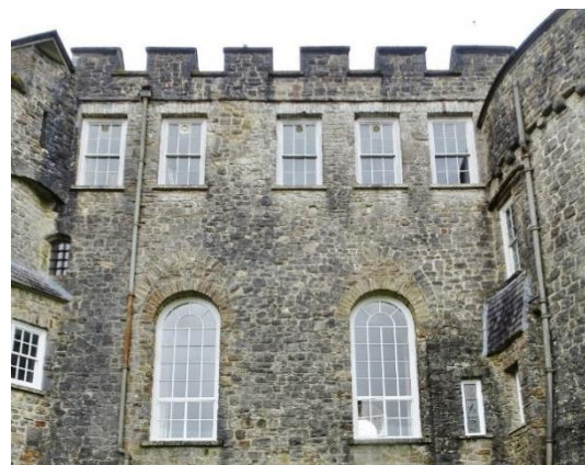
Fig. 173: North wall of central block, looking south, showing blocked chutes/sockets (beneath upper floor windows)
