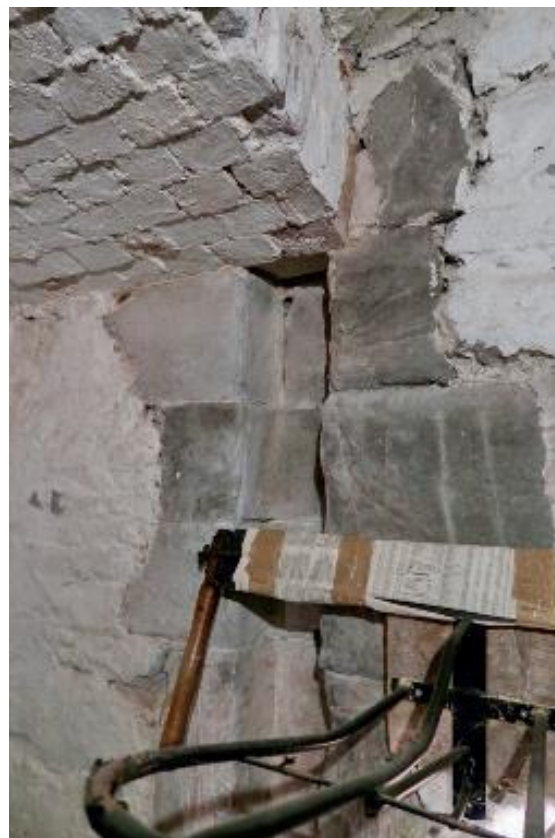
Fig. 33: Portcullis groove G2a-2 in passage south wall
