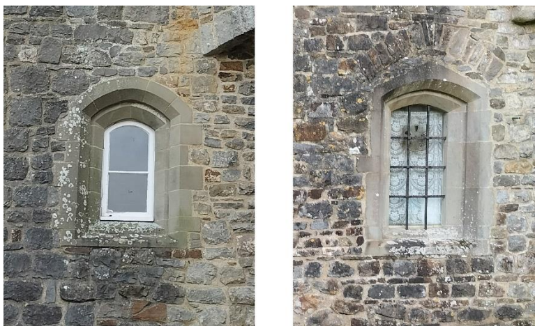
Fig. 231: 1960s double-chamfered surrounds: windows F13-2 and G9-4
