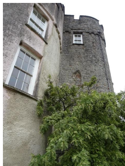
Fig. 122: External view of south gate-tower, showing blocked second-floor light S24-3 with medieval surround
