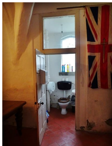
Fig. 73: North wall west opening G9-4, looking north
