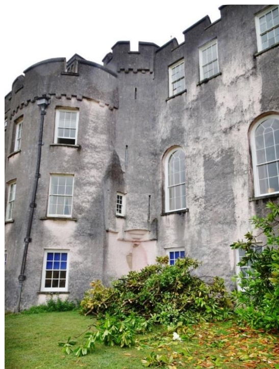
Fig. 110: External view of corbelling between the Southwest Tower and the Great Hall, carrying passage F20 and spiral stair SSC, looking northwest
