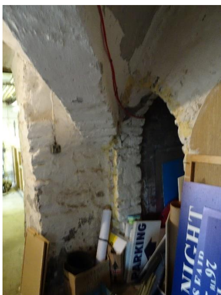
Fig. 64: Passage doorway G8-2, looking northwest
