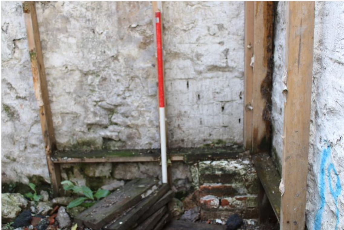
Photo 33: Possible remains of an earlier brick wall coming from the southwest wall (scale 1x1m).
