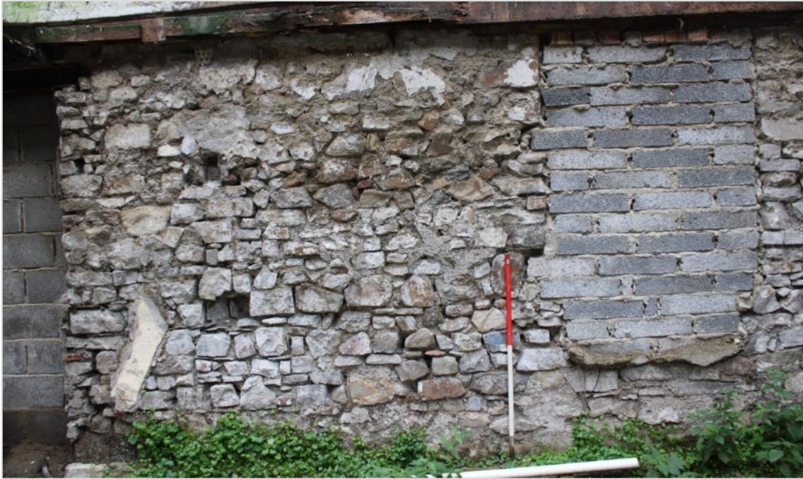
Photo 24: Northern section of the northwest wall with evidence of plaster, damage and a window infilled with breeze block (scale 1x1m).
