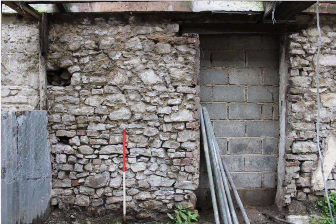
Photo 23: Western section of northwest wall. Stonework shows evidence for remodelling. Damage can be seen by missing stones and door has been infilled with breeze block (scale 1x1m).
