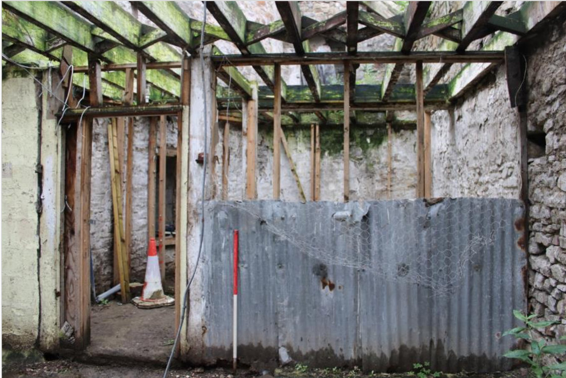
Photo 15: Section of partitioning timber studwork half covered in iron corrugated sheets (scale 1x1m).
