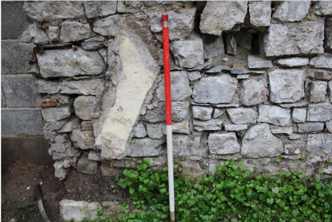
Photo 18 Large section of plaster on northwest wall (scale 1x1m).
