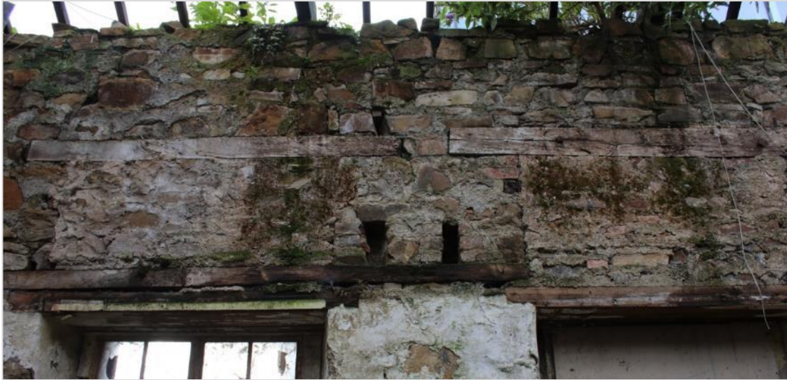
Photo 40: Southeast wall infilled with stone. Pockets for timbers present and a long timber sits above the open window.
