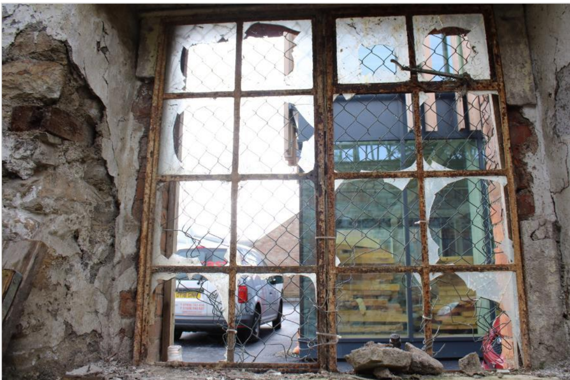
Photo 22: Open window on southeast wall; metal with modern wire. Glass is still intact.
