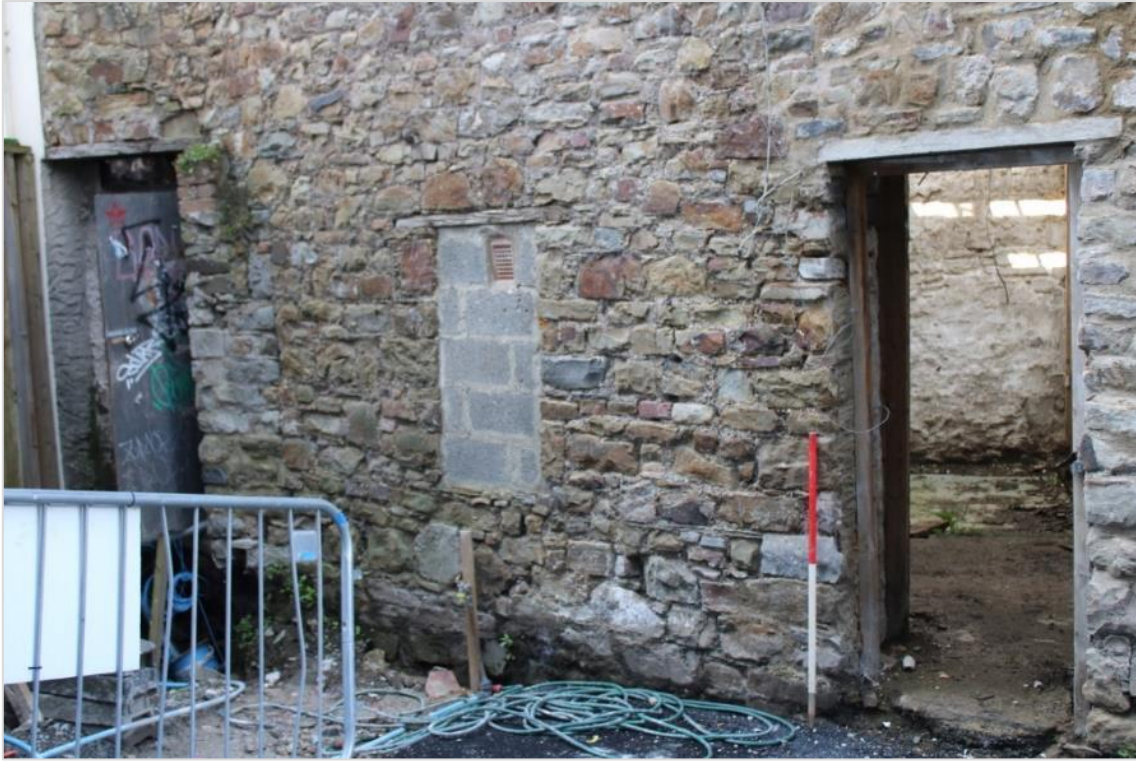
Photo 5: View northwest of doors on south and southeast walls and infilled window on south wall (scale 1x1m).
