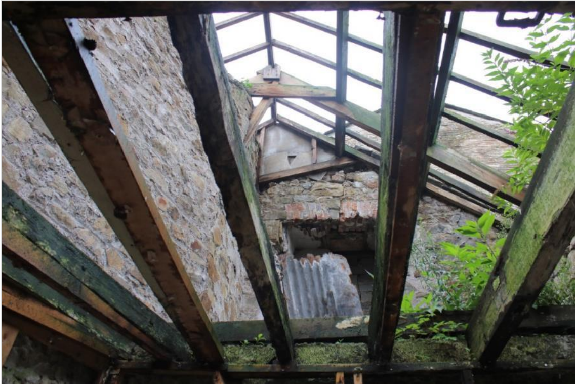
Photo 35: Tapered southern wall. Truss has been cut and built into stone wall.
