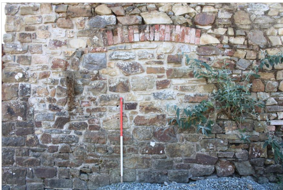
Photo 13: The northern window on the northwest wall which was not within the lean-to. Window infilled with like-for-like stone and a cement mortar. The original brick arch can be seen (scale 1x1m).
