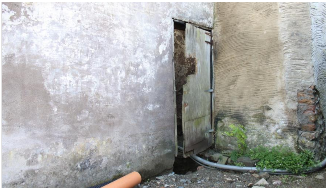
Photo 10: Southern door on northwest wall. Still in use and was part of the lean-to. The door has a timber frame.
