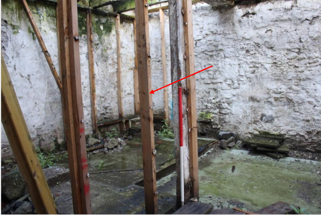
Photo 26: Western view of small room, divided by a timber stud wall (red arrow), the result enhanced by the in situ concrete slab being at different heights (scale 1x1m).
