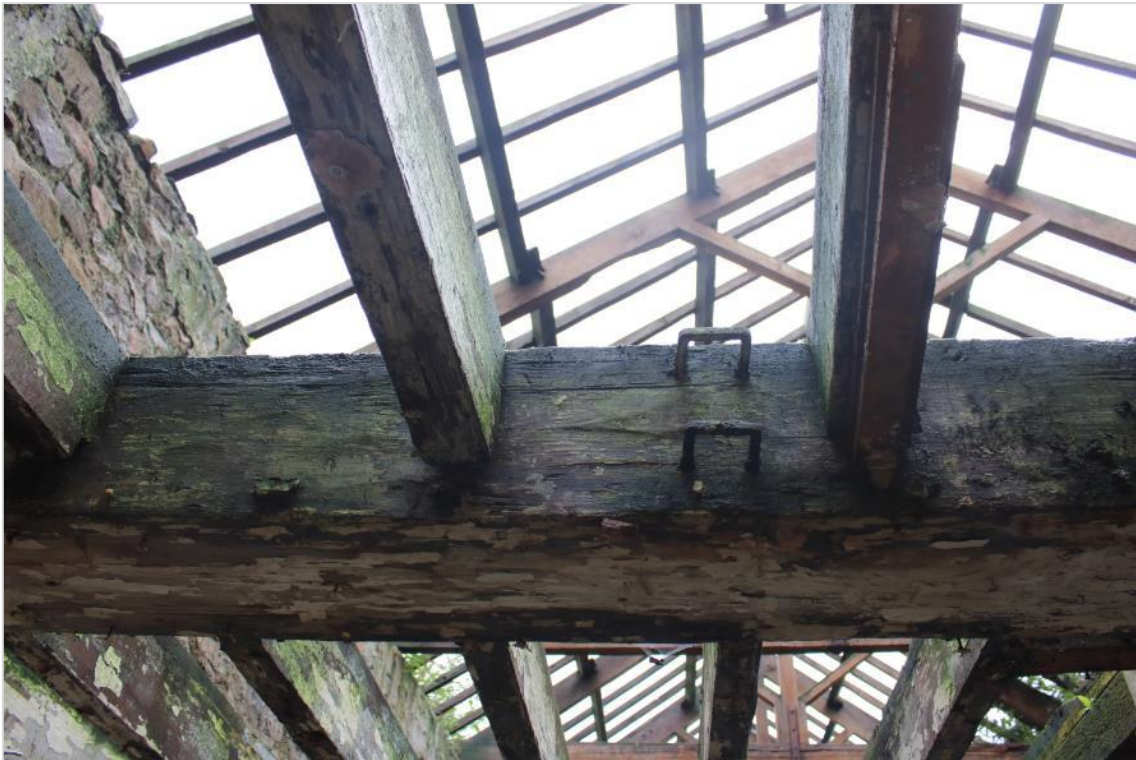
Photo 36: Example of metal work in the timber for the roof and floors, possibly relating to the foundry.
