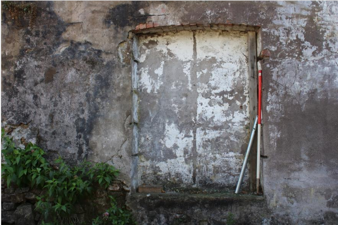
Photo 12: Infilled window on northwest wall. Covered in render suggesting it was infilled when the lean-to was in use. A brick arch can be seen under the render (scale 1x 1m).
