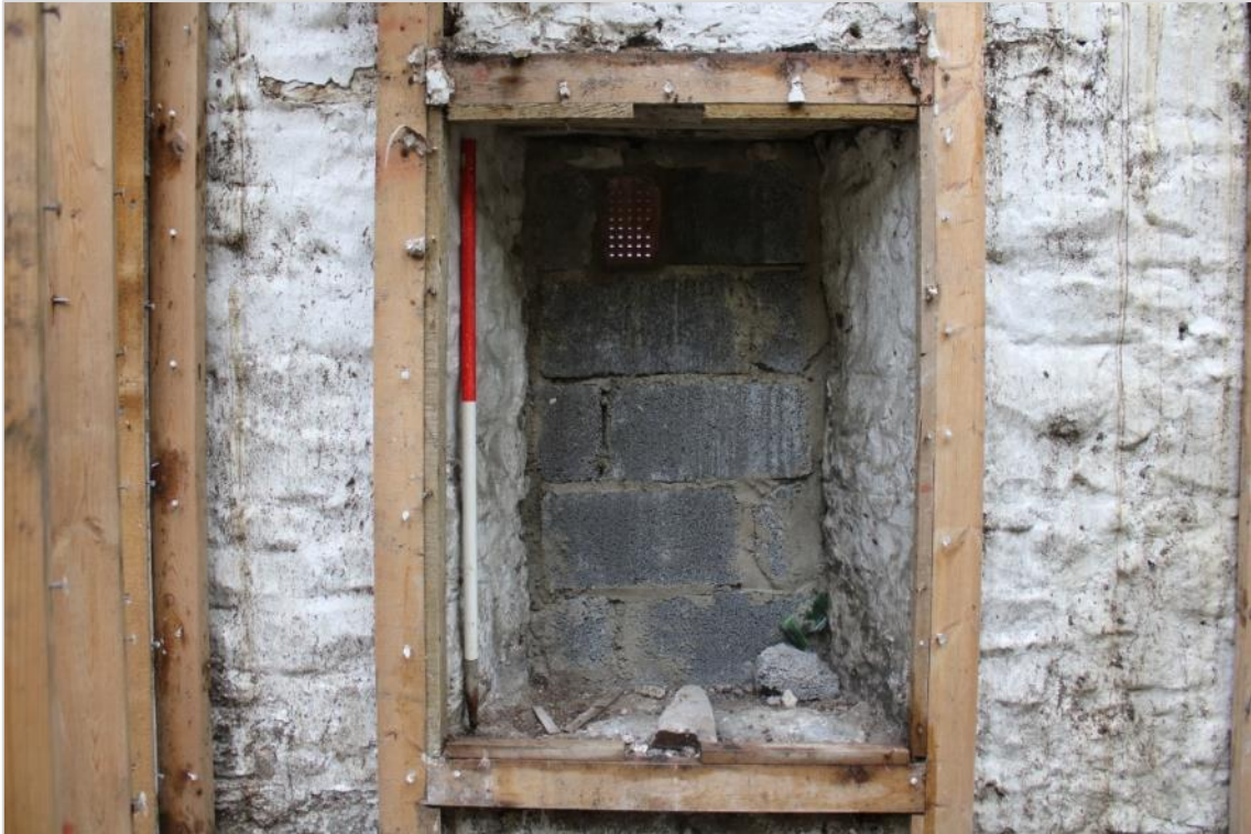
Photo 29: Window in the small room. Sides taper in. Breeze block infill and brick air vent (scale 1x1m).
