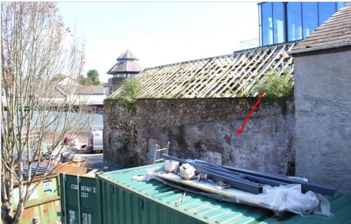
Photo 9: Eastern view of render from lean-to on the northwest wall (indicated by red arrow). Exposed single duo pitch roof.
