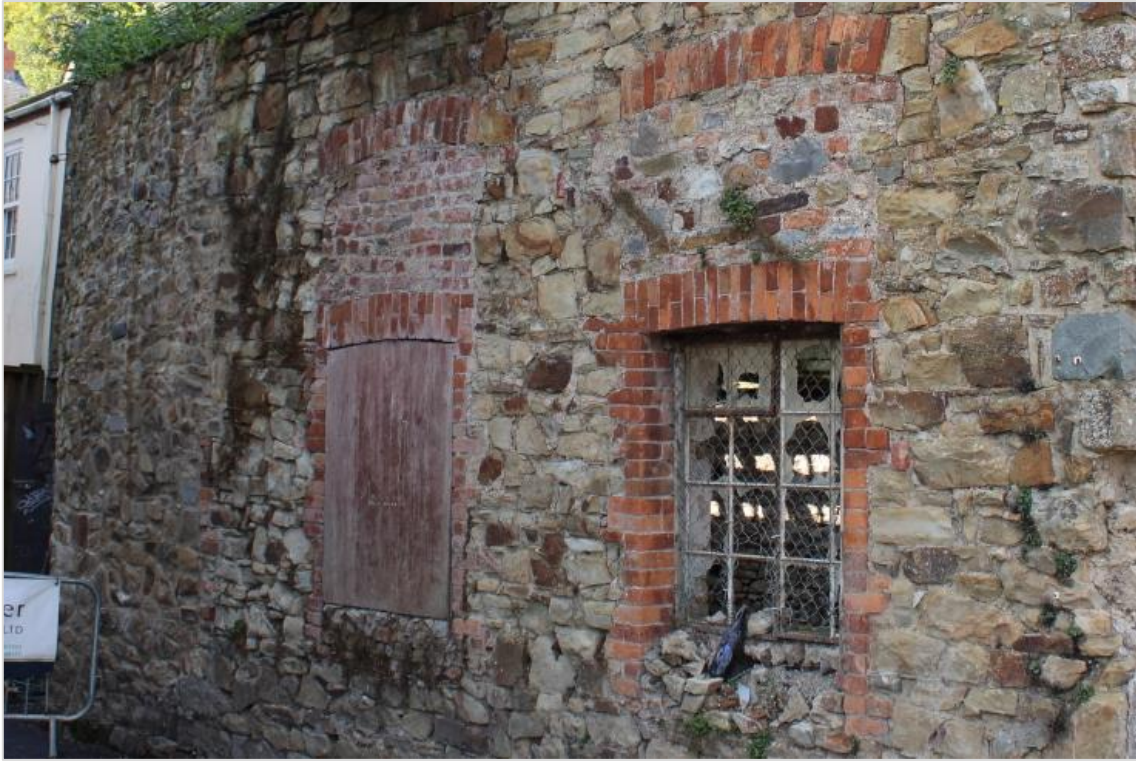
Photo 6: Windows on southeast wall. One remains open and has glass intact. Both windows have evidence of an infilled window above, one with brick (to the left) and the other (to the right) stone.
