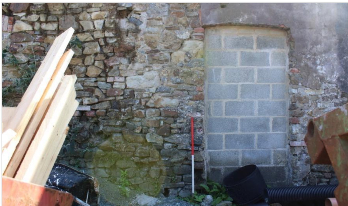
Photo 11: Southeast view of door in the lean-to. Infilled with breeze block. Evidence of a stone arch under render (scale 1x 1m).
