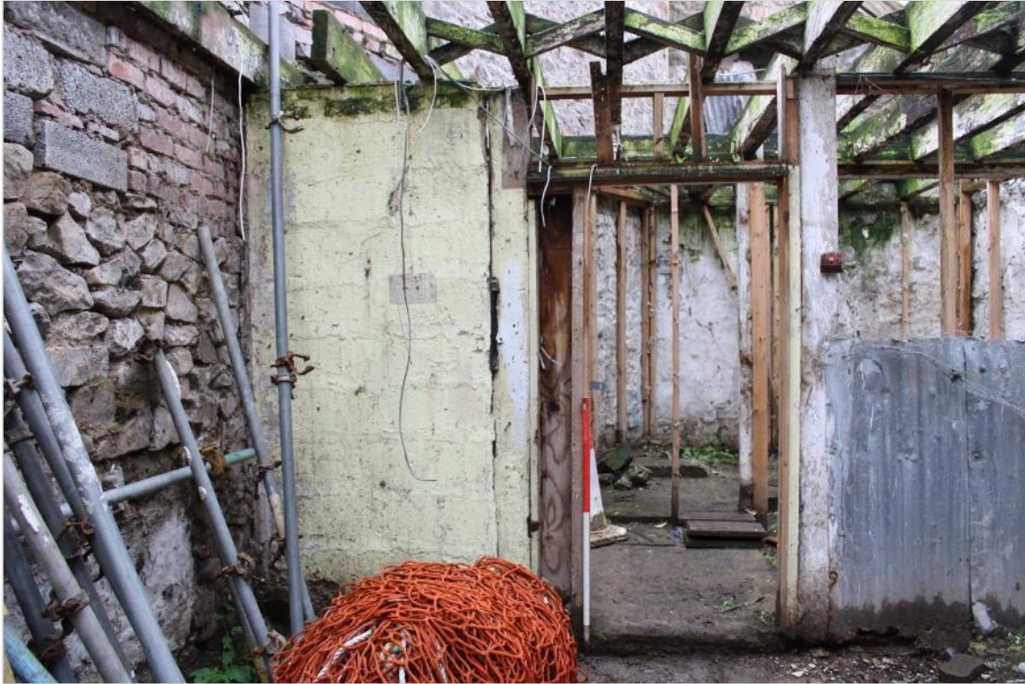
Photo 14: Breeze block section of wall which partitions the two interior ground floor rooms. The doorway is timber framed (scale 1x1m).
