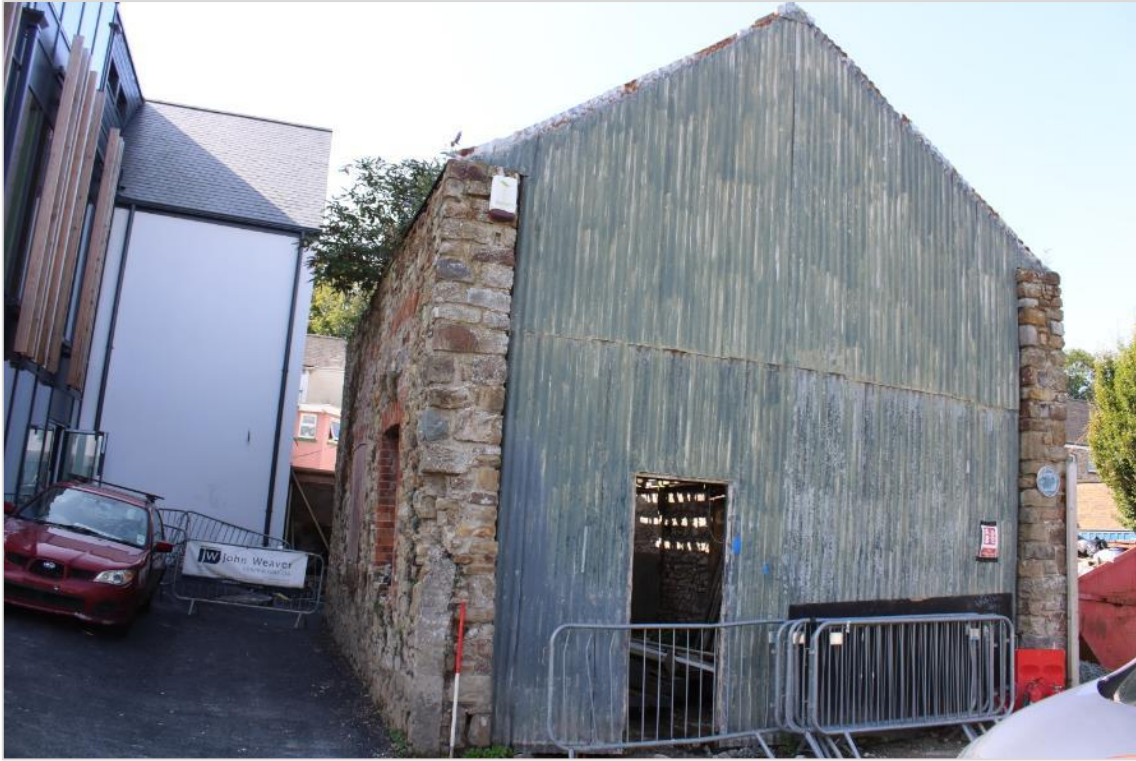
Photo 7: West facing view of northeast wall. The edges have modern stone facing and northeast wall replaced with corrugated iron sheets on timber studwork (scale 1x 1m).
