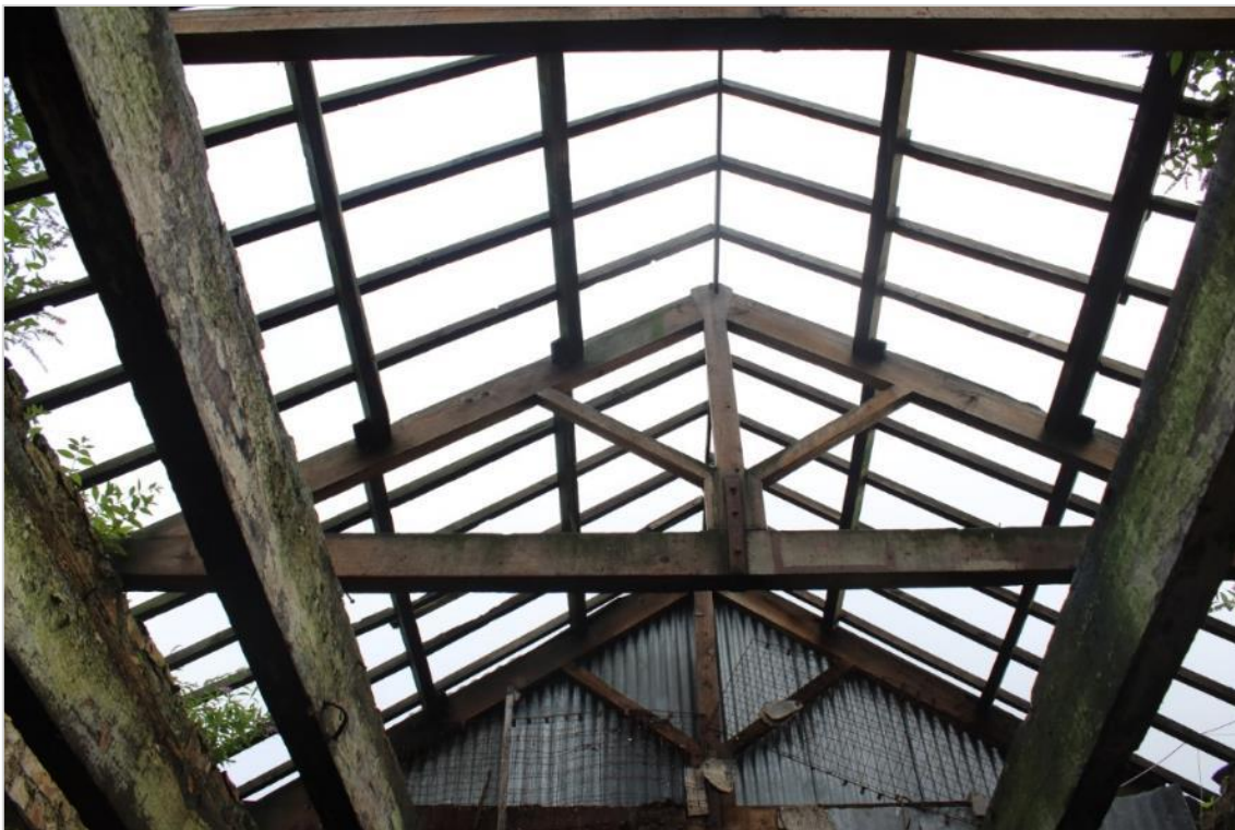
Photo 34: King post trusses supporting a duo pitch roof.
