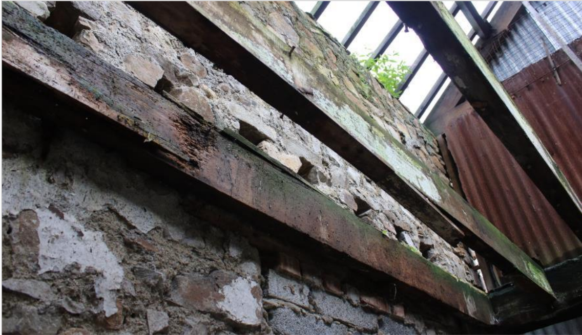
Photo 38: Sockets on the southeast and northwest walls. Evidence for an earlier floor level and different joist direction.
