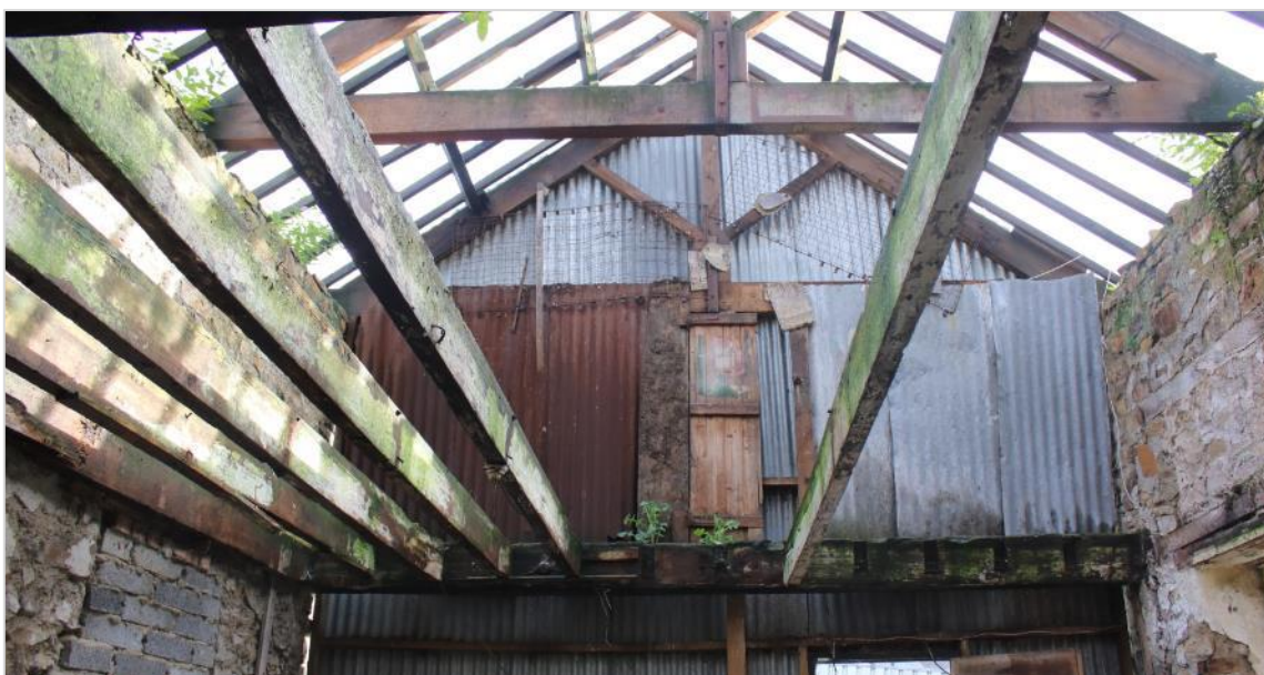
Photo 41: First floor of northeast wall with earlier central door with a timber frame.
