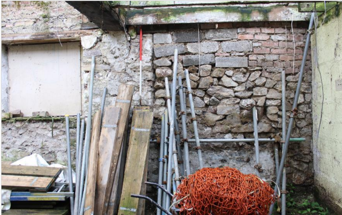
Photo 20: Southern section of southeast wall. Evidence of alterations using brick, stone and breeze block. A clear divide between the original stonework and new can be seen (scale 1x1m).
