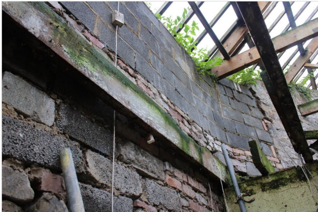
Photo 39: Southern section of southeast wall and part of the southern wall. At first floor level, breeze block and brick were used.
