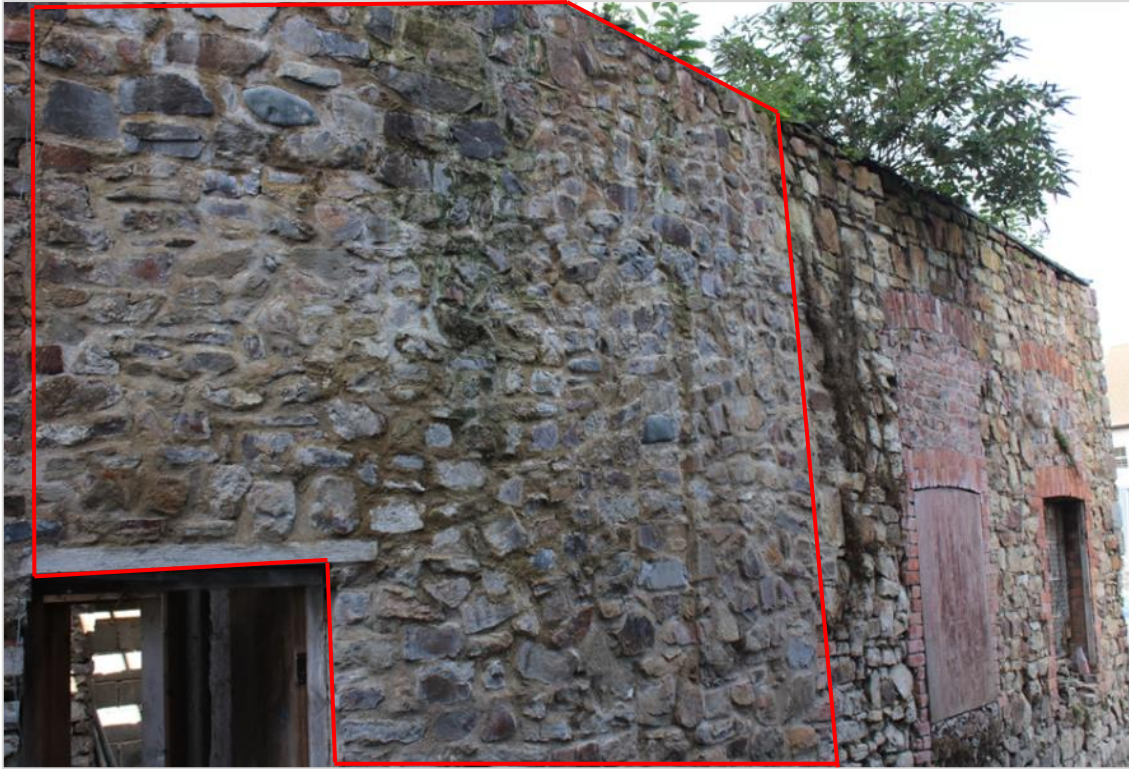
Photo 3: 4m panel of rebuilt masonry on the southeast wall.
