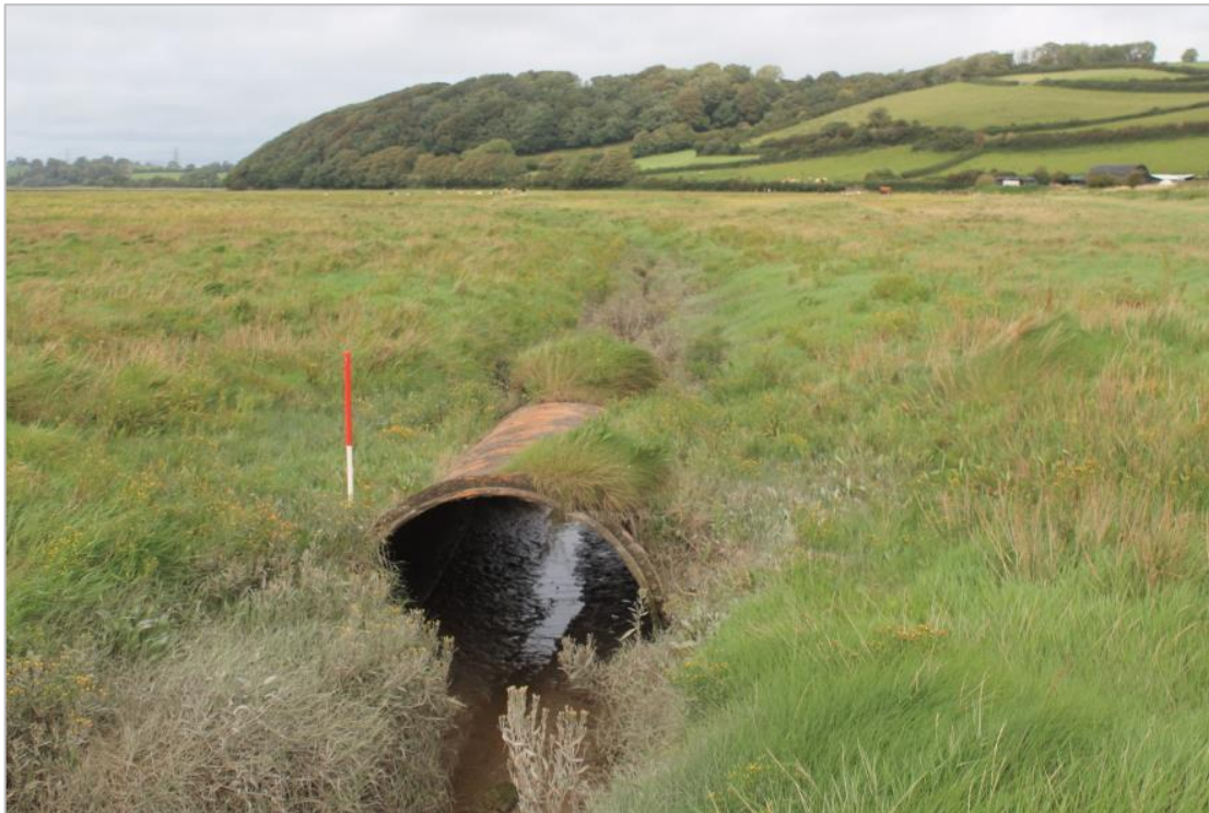
Photo 27: View north, showing a cast iron cylinder bridging a small stream to the west of the flood defence bank.
