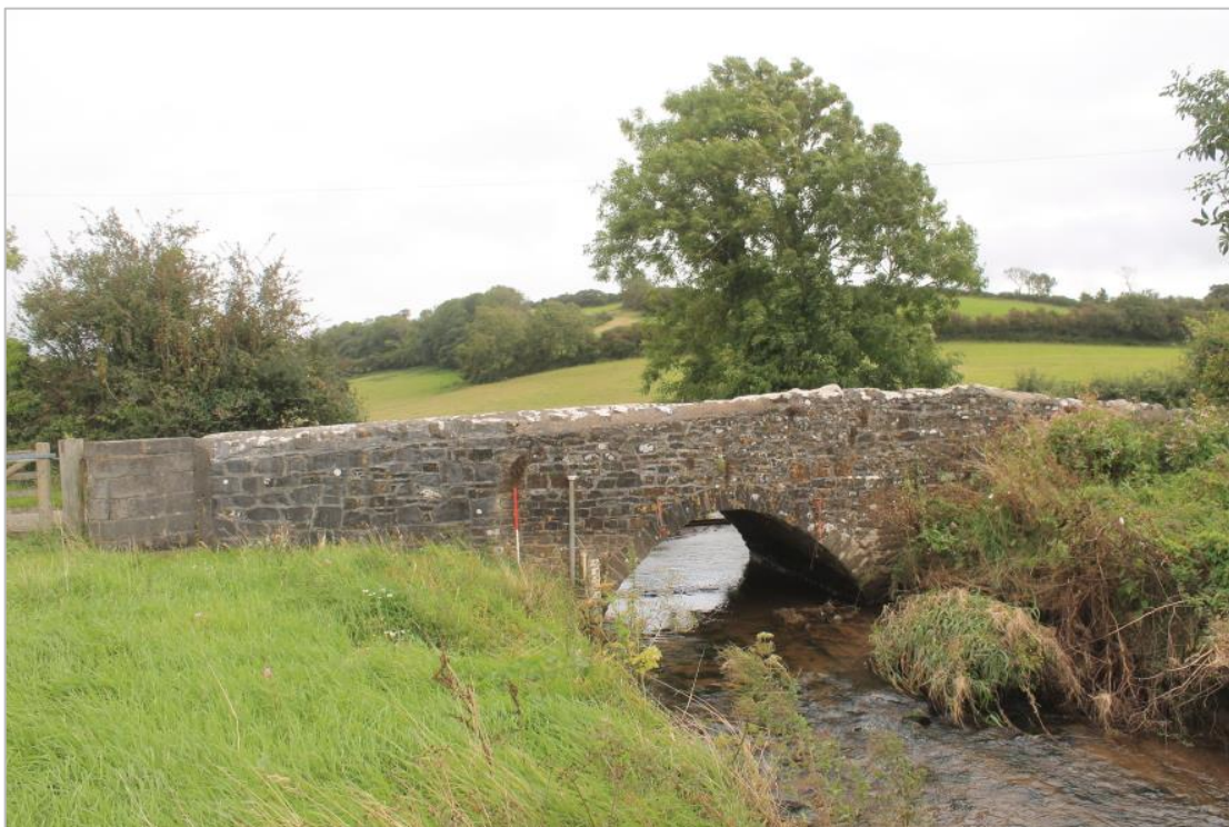
Photo 15: Pont y Moche bridge, showing a change in the stonework of the western wall, either side of the 1m scale. View east.
