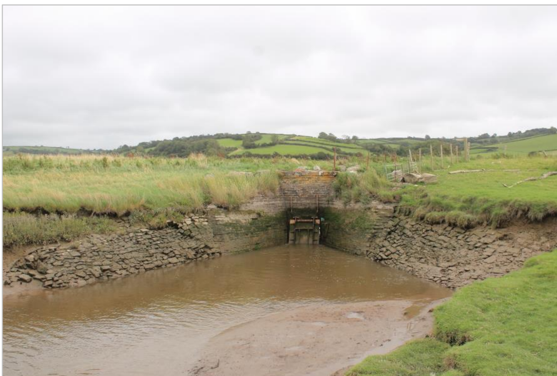
Photo 25: View east, showing the iron sluice gate hung within the stone-revetted V-shaped opening in the flood defence bank. Note a pair of iron runners mounted on the wall above the gate.
